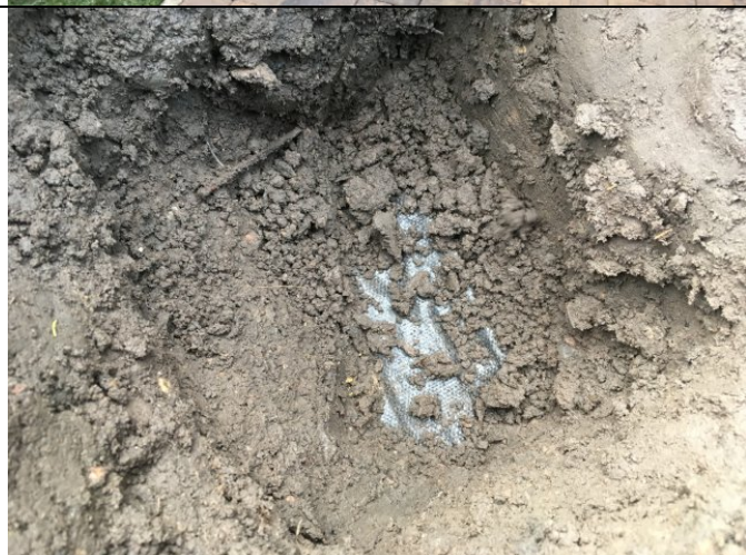
Photograph 2: View of soil in capping layer excavation in front garden of Plot 31 with geotextile membrane visible.
