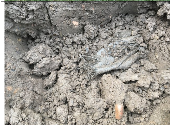
Photograph 5: View of soil in capping layer excavation in rear garden of Plot 31 with geotextile membrane visible.
