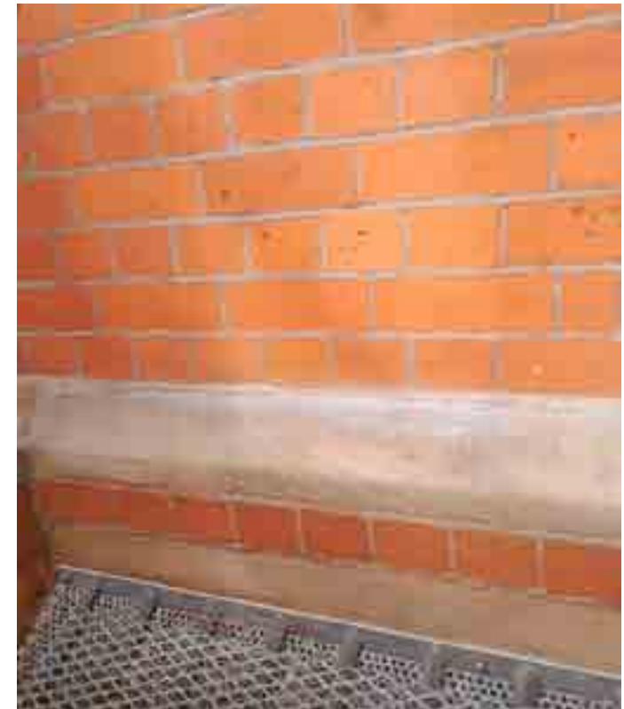
repointing stone string
