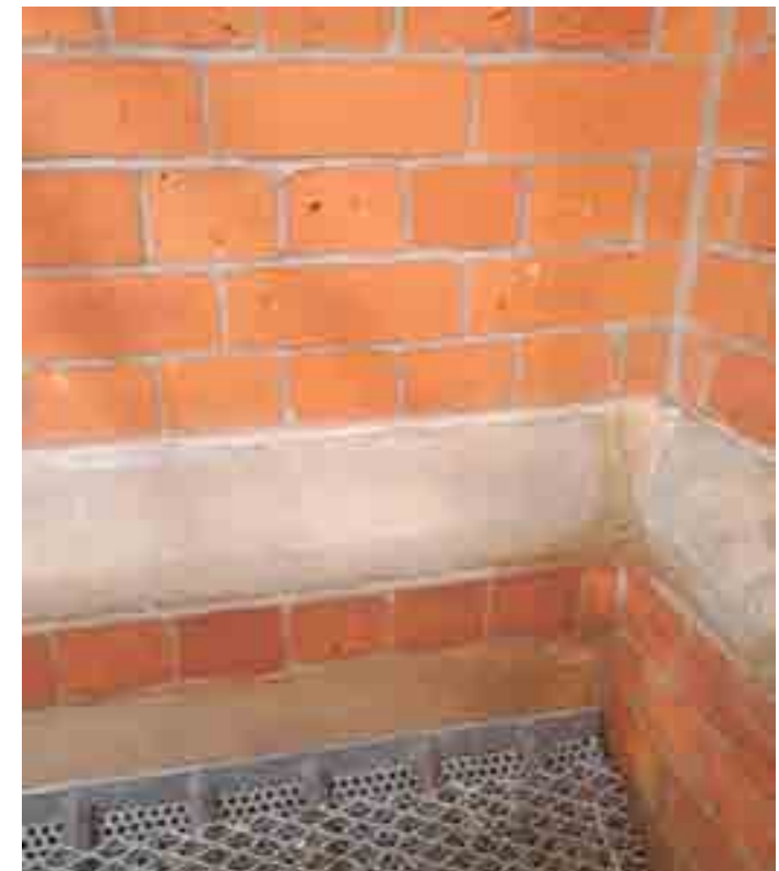
repointing of stone string internal corner
