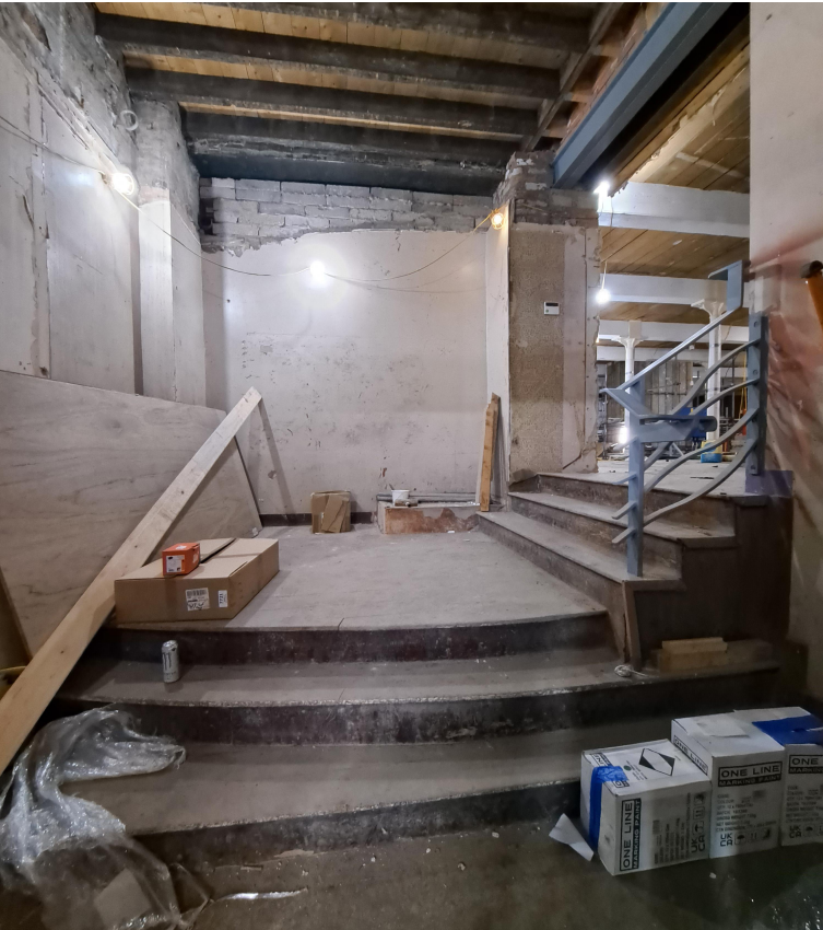
1. Timber steps to be removed
