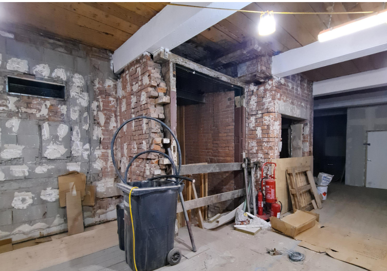
4. Timber frame + Lift shaft
