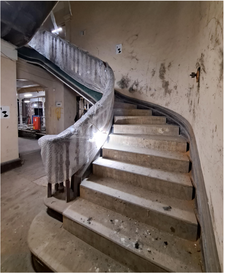
5. Mains tair to be retained and repaired
