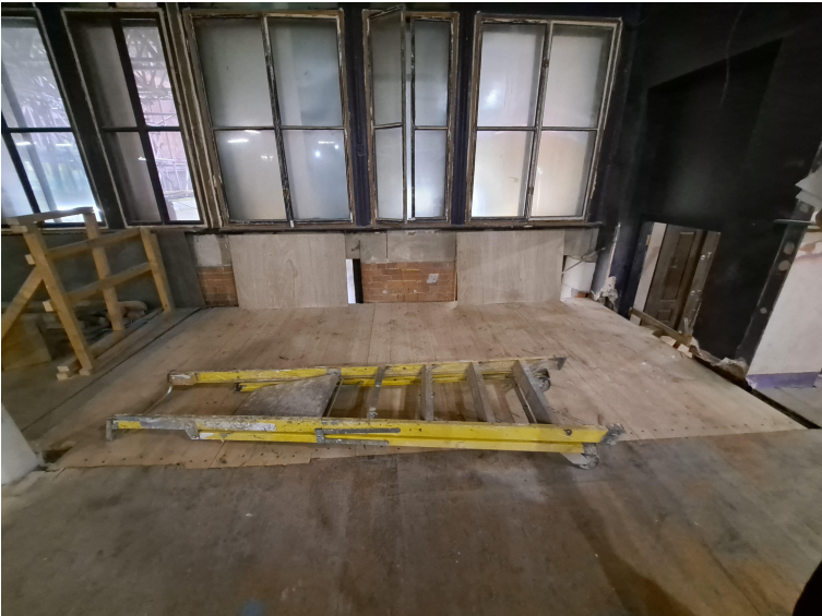
2. Floor infill + existing windows
