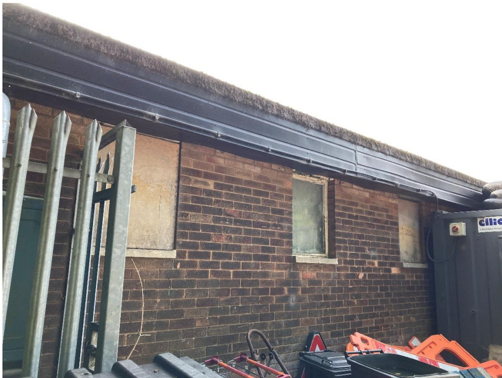
Image 02 – Ladder Access Location Nr.1
