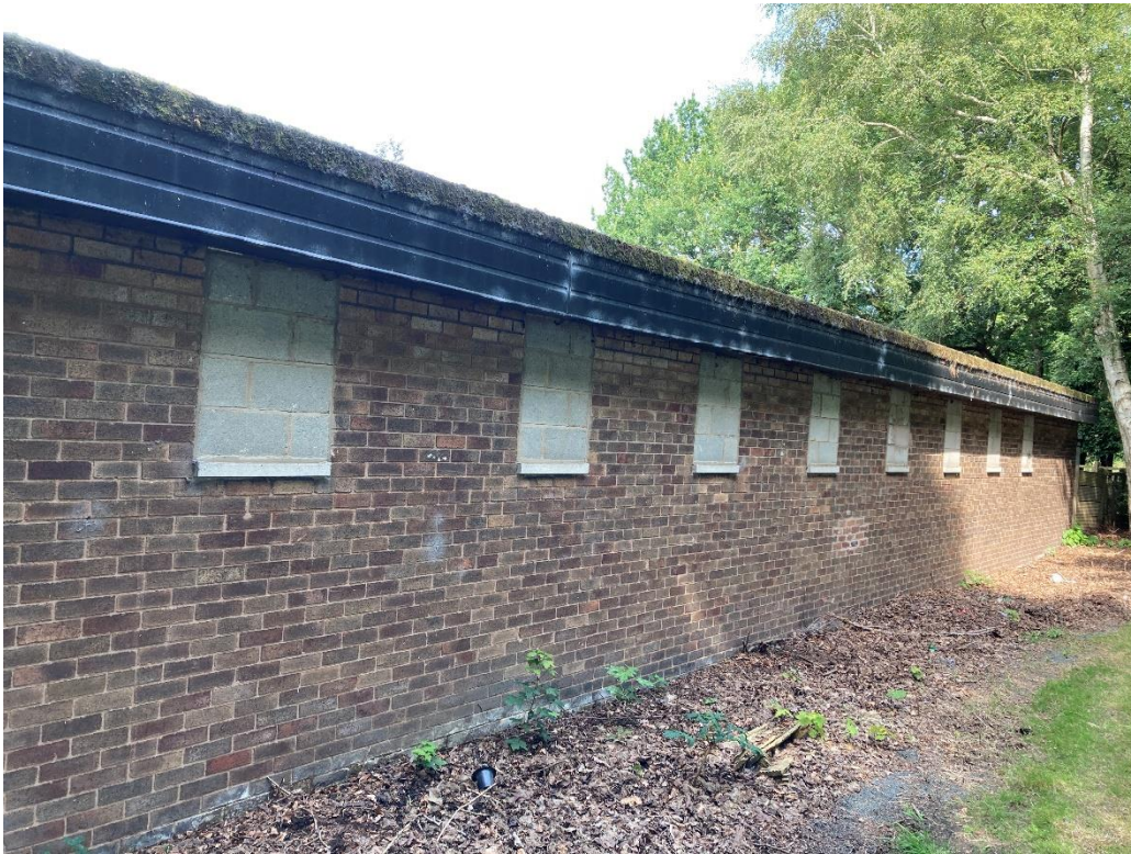
Image 03 – Outer wall to receive low level pipework and cable tray protrusions
