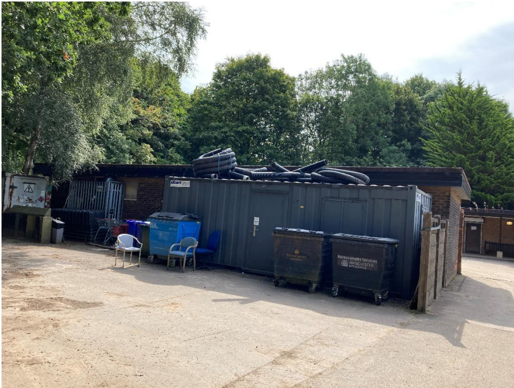
Image 01 – Ladder Access Location Nr.1
