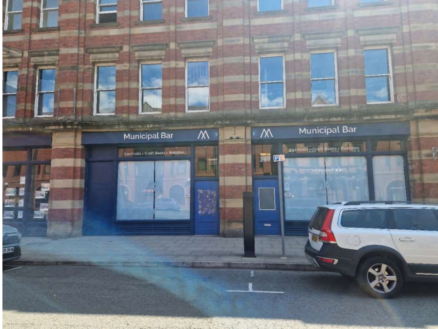
Image 1: Present Shopfront Elevation, Deansgate, Manchester
