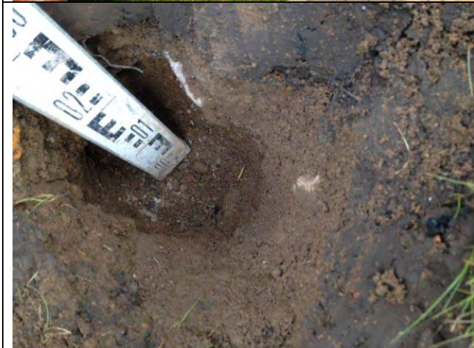
Photograph 35: View of soil in capping layer excavation in front garden of Plot 15 with geotextile membrane visible.
