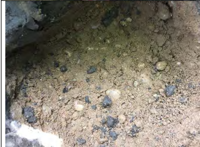
Photograph 5: View of soil in capping layer excavation in front garden of Plot 10 with MOT break layer visible.
