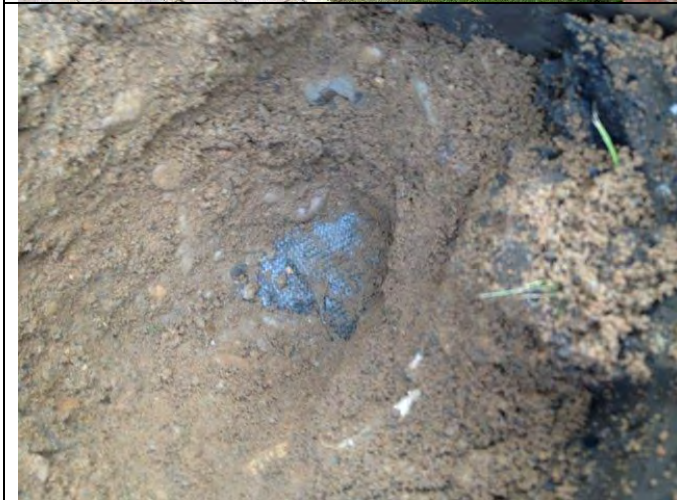
Photograph 29: View of soil in capping layer excavation in front garden of Plot 14 with geotextile membrane visible.
