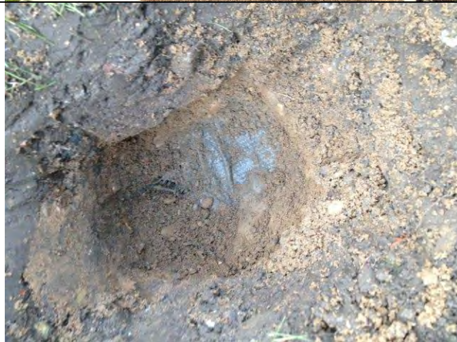
Photograph 41: View of soil in capping layer excavation in front garden of Plot 16 with geotextile membrane visible.
