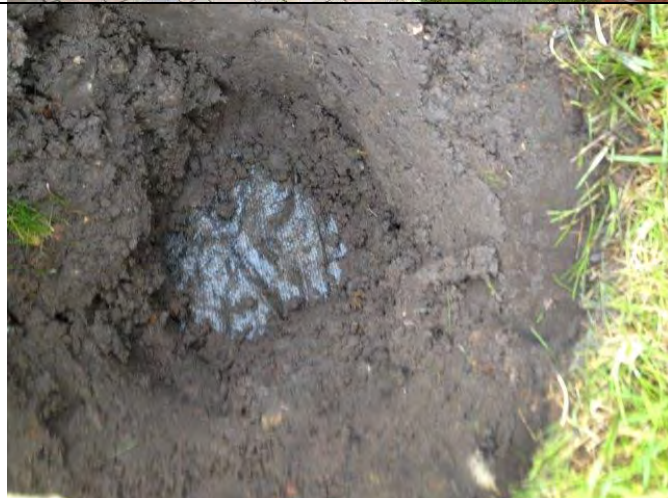
Photograph 17: View of soil in capping layer excavation in front garden of Plot 12 with geotextile membrane visible.
