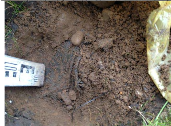
Photograph 11: View of soil in capping layer excavation in front garden of Plot 11 with geotextile membrane visible.
