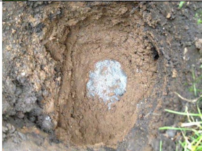
Photograph 47: View of soil in capping layer excavation in front garden of Plot 17 with geotextile membrane visible.
