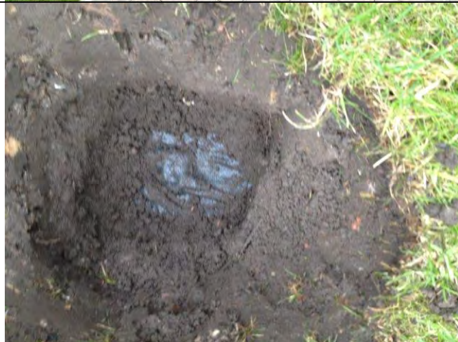
Photograph 23: View of soil in capping layer excavation in front garden of Plot 13 with geotextile membrane visible.
