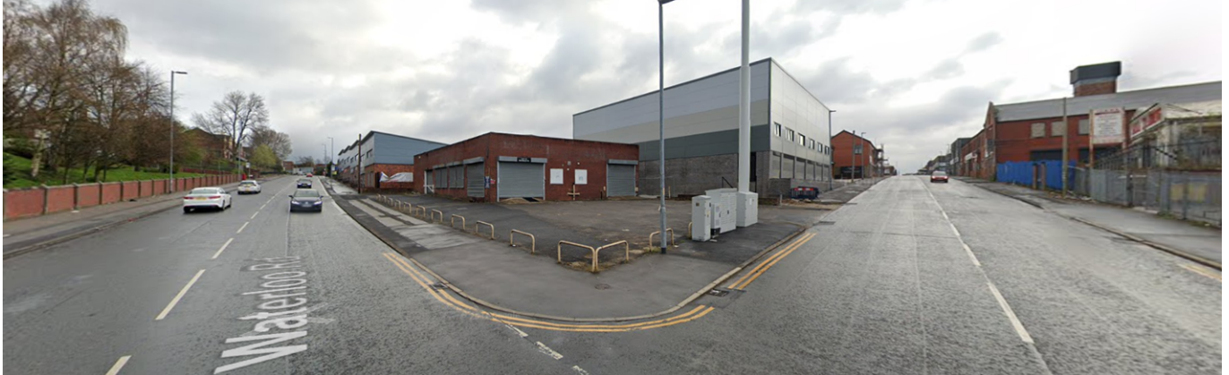
Figure 4. Previous boundary treatment (April 2021)
