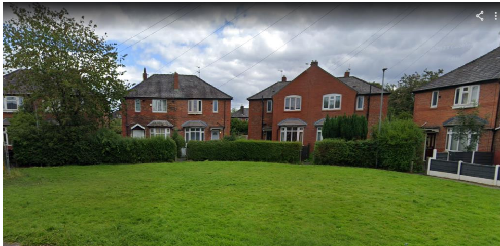
Fig 3 View of front elevation of number 16 Anfield Road
