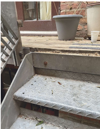
Fig. 07 Photo showing existing timber boards at the top of the stairs, and also the existing aluminium checker plate stair treads.
