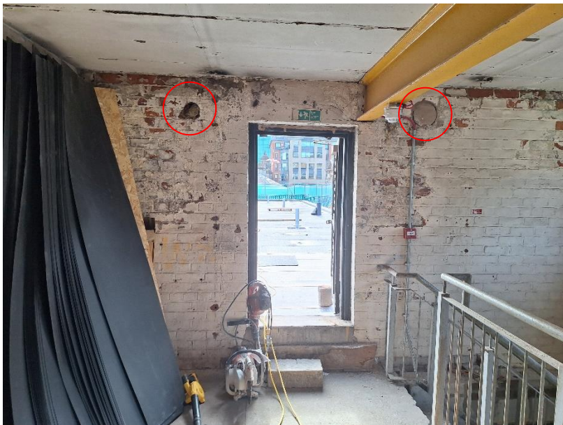
Figure 11 Showing Sealed Holes in Brickwork
