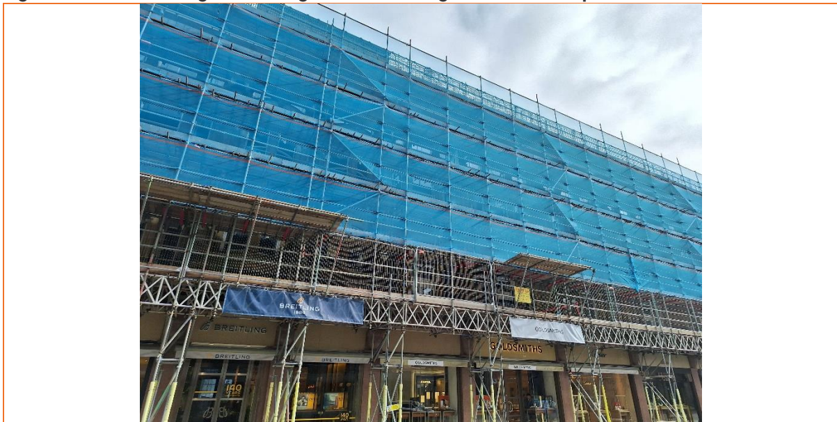
Figure 2 Showing Scaffolding and Bird Netting on Southern Aspect
