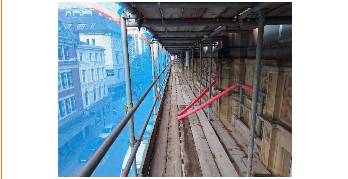
Figure 5 Showing Scaffolding and Bird Netting
