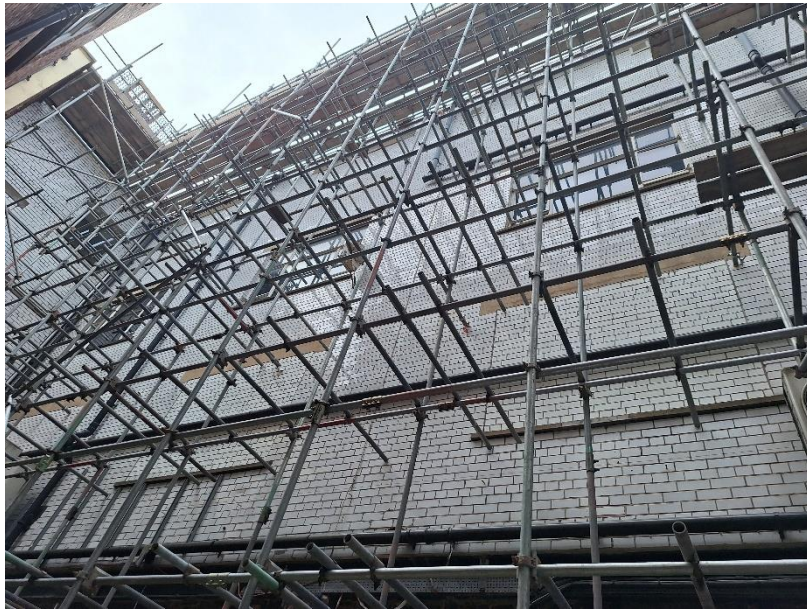
Figure 3 Showing Scaffolding on Northern Aspect
