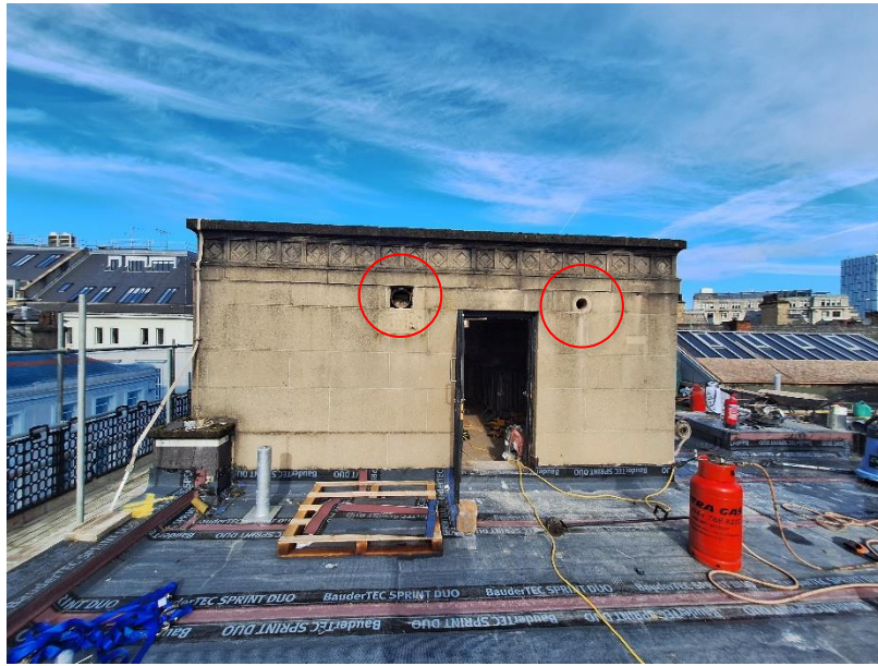
Figure 10 Showing Flat-Roofed Structure
