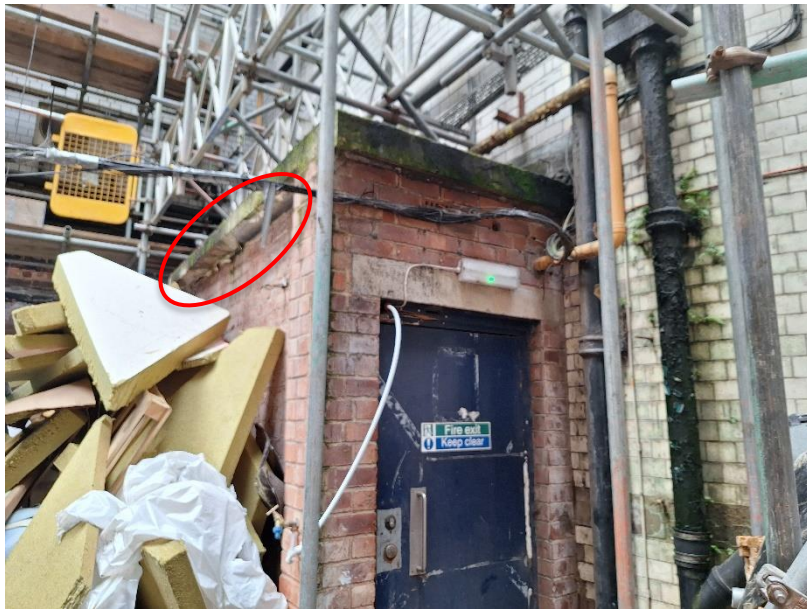
Figure 4 Showing Fire Exit
