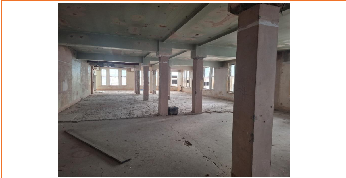
Figure 12 Showing First Floor Internals
