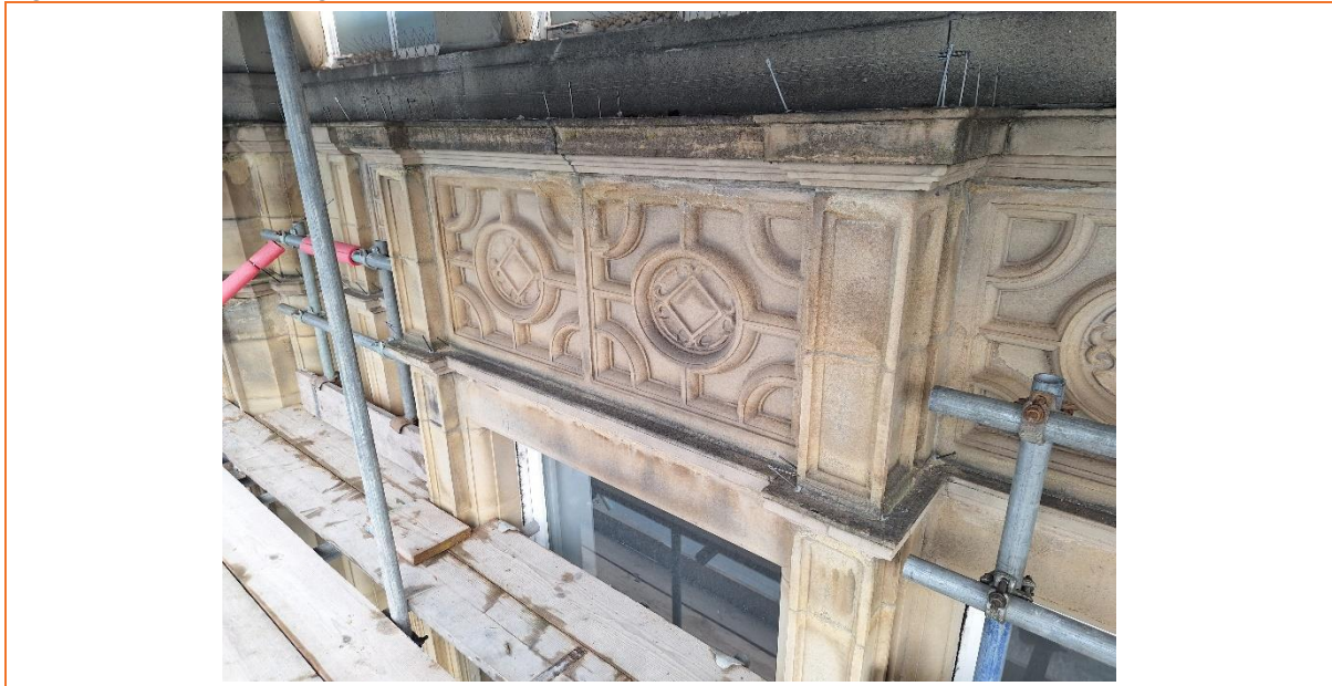
Figure 7 Showing Stonework Facade
