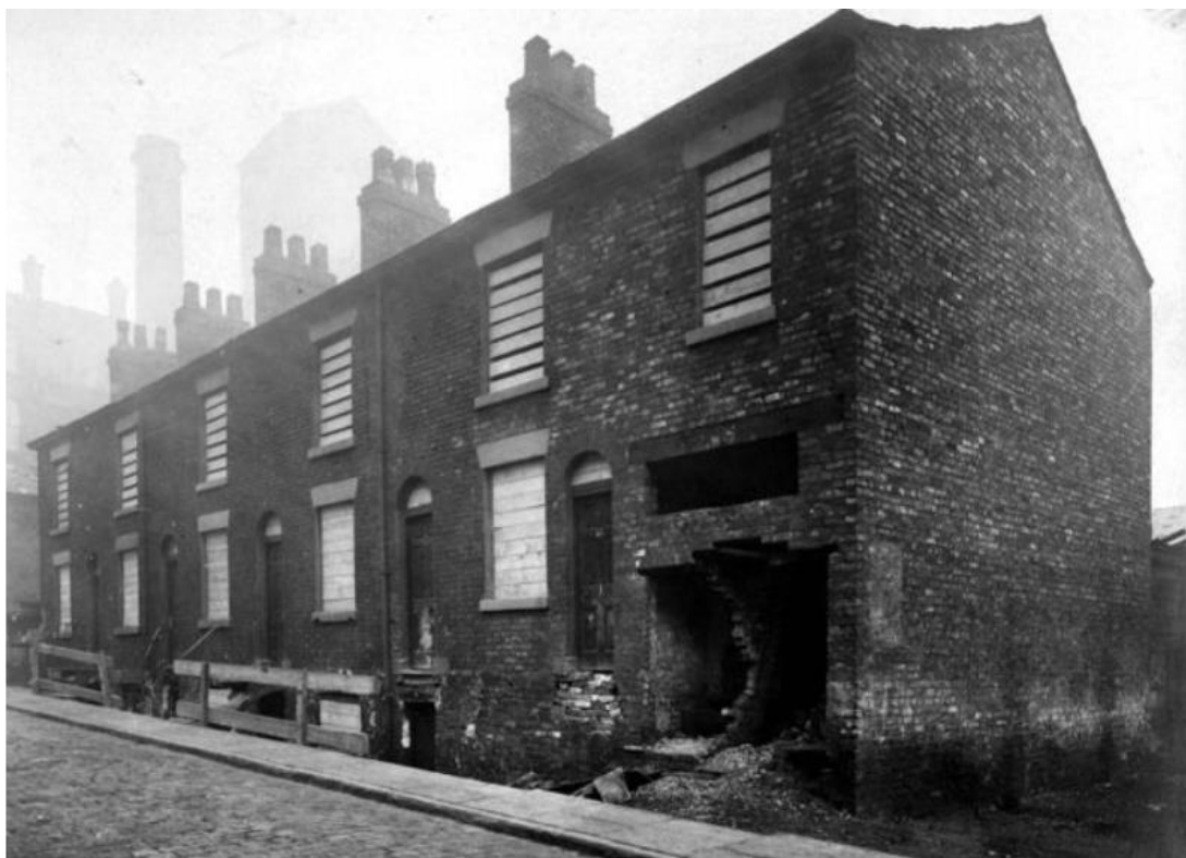
Plate 15: Nos. 55-63 Poland Street, Ancoats, 1908, note the chimney of the City Corn mill, rear of shot (m10403)
