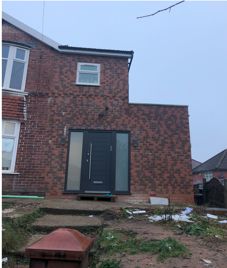
Figure 1, Applicant site and built two storey front extension
