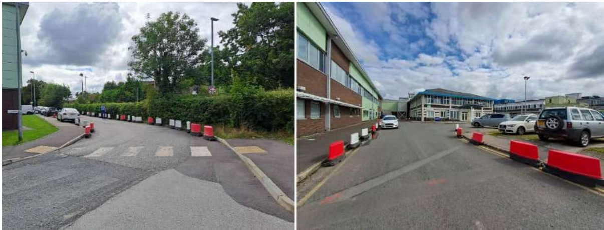
Figure F: Hospital Western Access Road to the NW and SE of the Site
