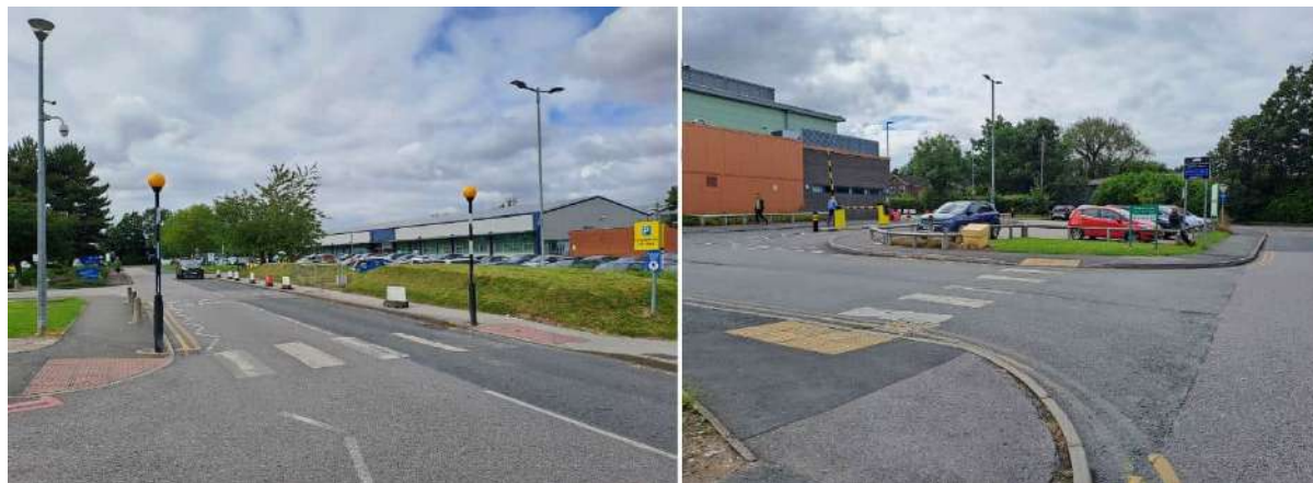
Figure K: Pedestrian Crossing Facilities on Southmoor Road
