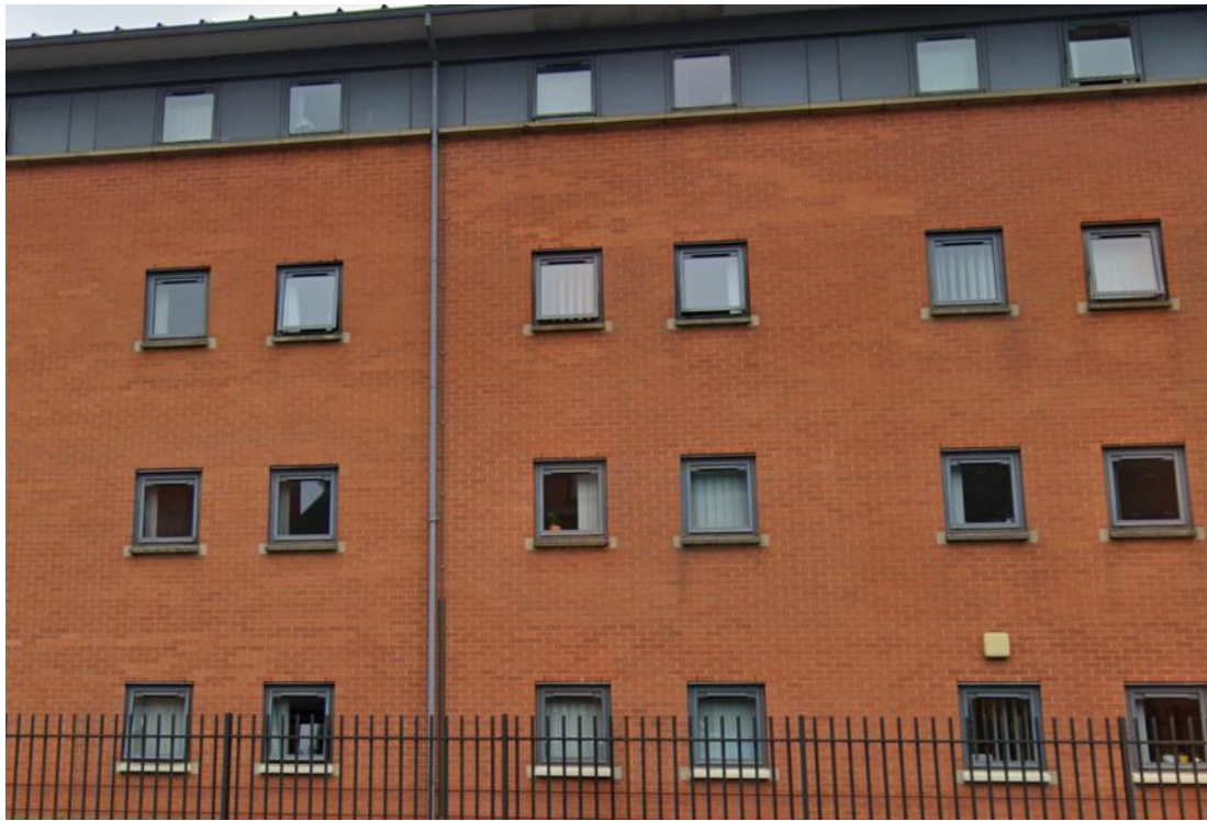
Representative view from Upper Cambridge Street. All brick work, windows, cladding and other features are tight with no visible gaps or cavities. No bat potential roost features were observed.
