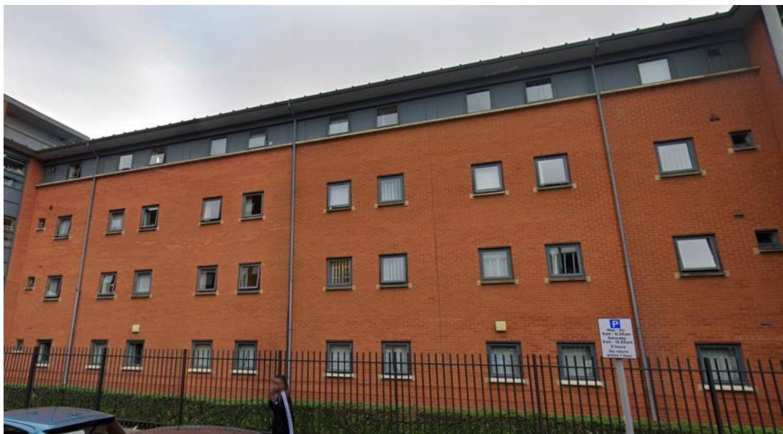
Representative view from Lower Chatham Street. All brick work, windows, cladding and other features are tight with no visible gaps or cavities. No bat potential roost features were observed.
