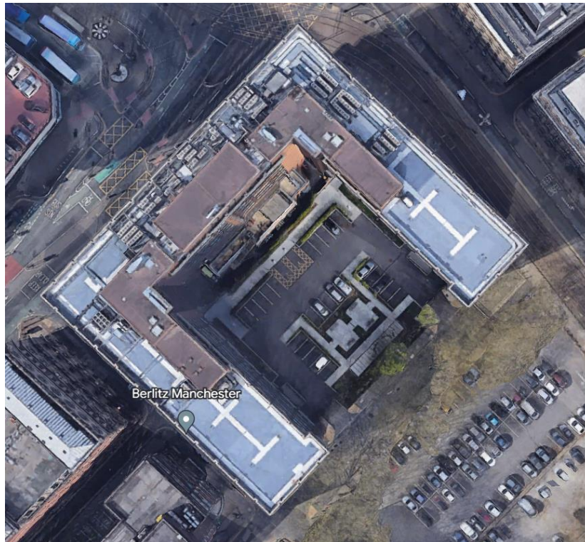
Typical Location of existing Mechanical Plant
