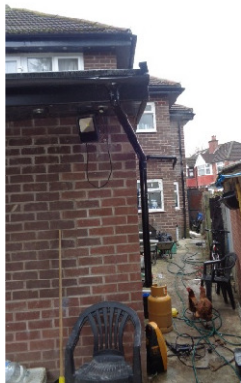
Gable Elevation to Application Property.
