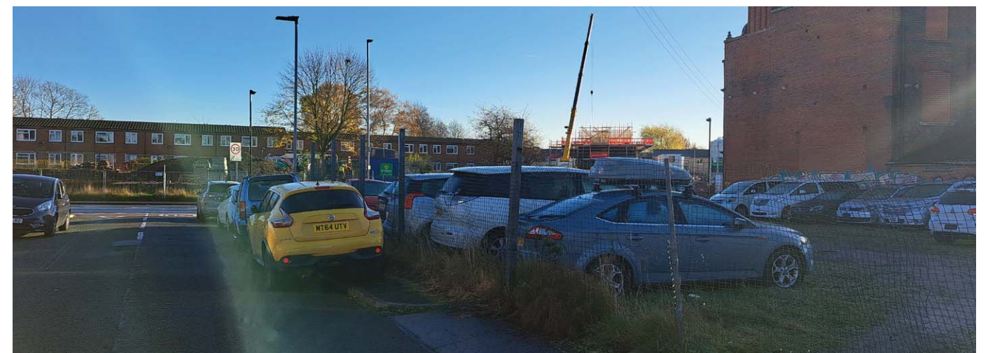
Lack of appropriate pavement along Cockcroft Street
