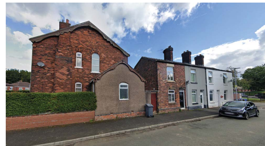
Photographic Survey - Cockcroft Street
