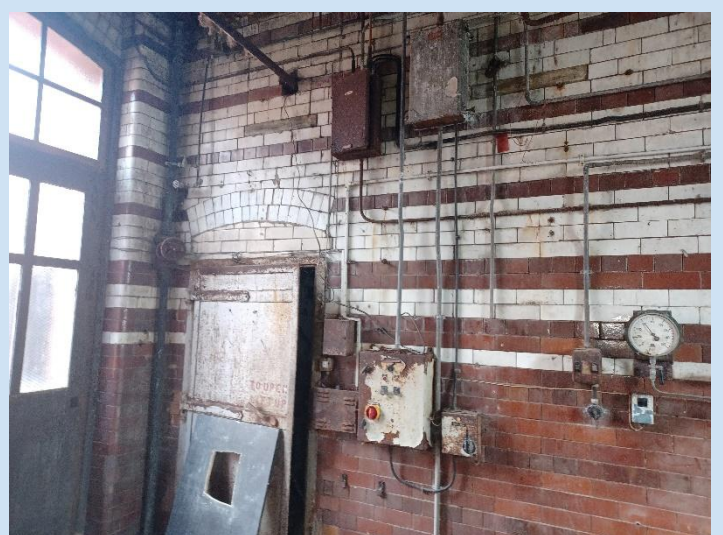
0/B02/GF-001-chlorination plant – Example of the electrics to be removed
