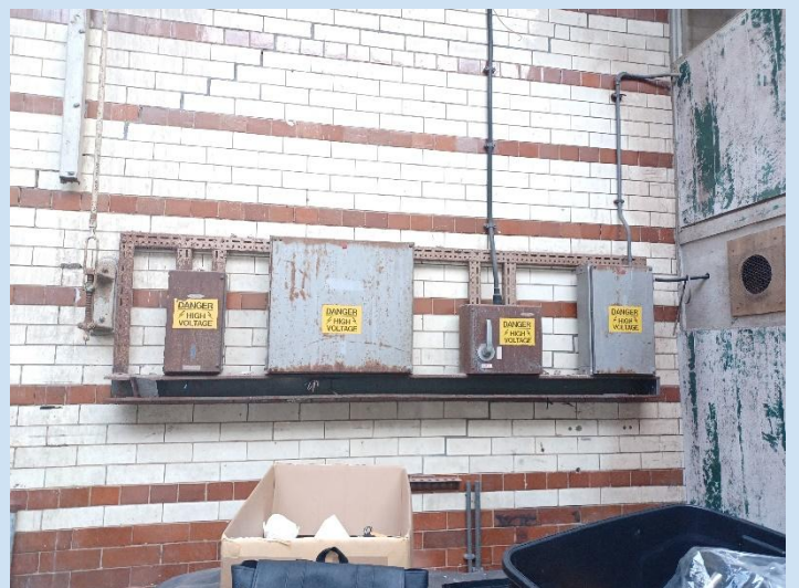
0/B03/GF-001-Laundry – Electrics to be removed
