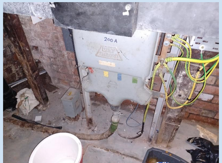
-1/B01/B1-003-electrics – Electric intake to electrics to be removed
