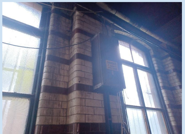
0/B02/GF-001-chlorination plant – Electrics to be removed
