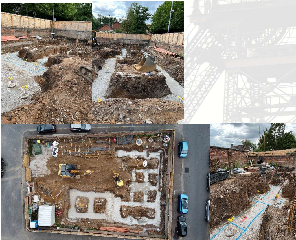
August 2023 – Piling complete- foundations poured.
