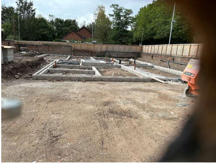
September 2023 Brickwork – DPC in progress
