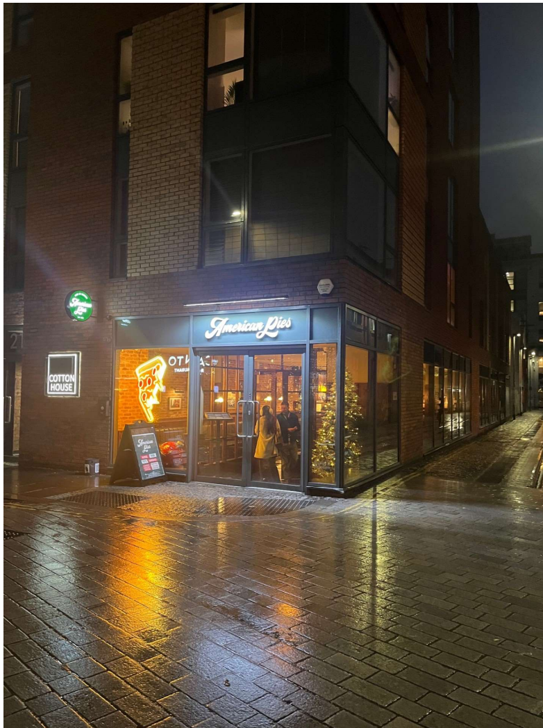
Site with signage in situ (December 2024)
