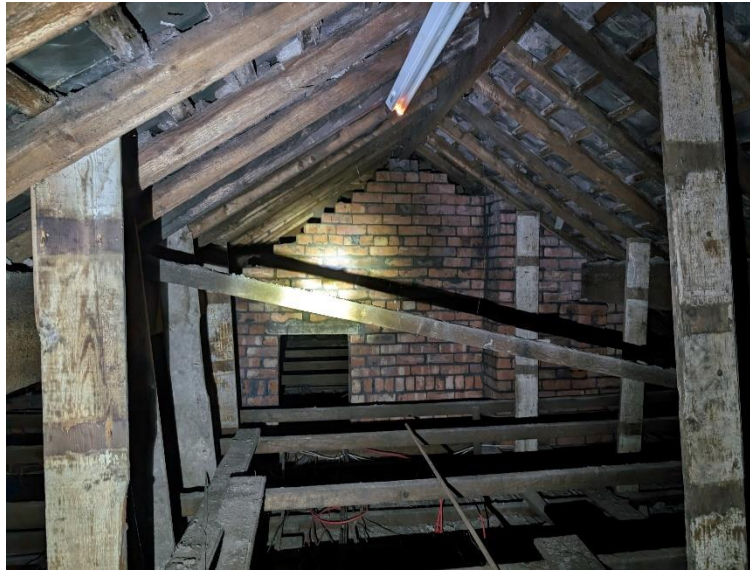
PLATE 3 SHOWING THE LOFT VOID
