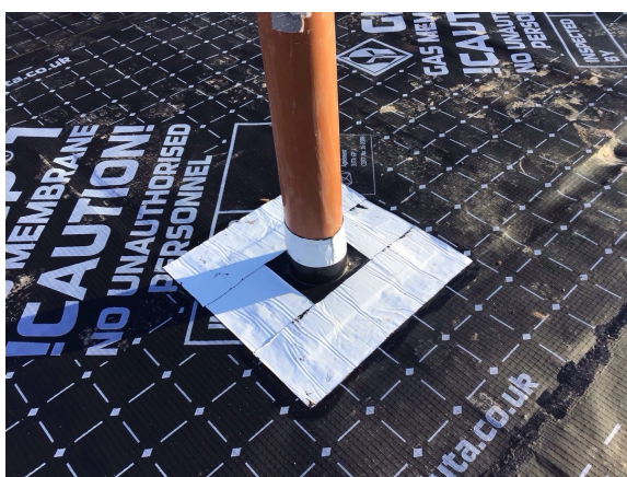
Detailed pipe penetration
