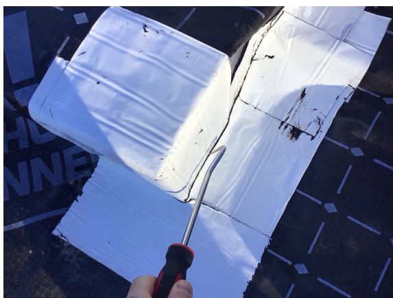
Testing threshold detailing
