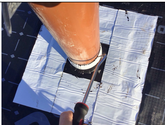
Testing pipe detailing
