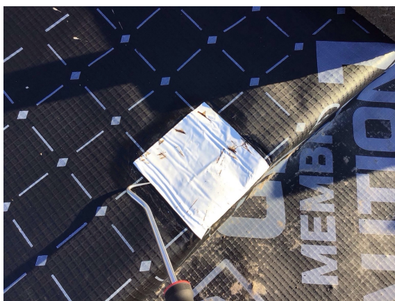
Testing installers CQA patch repair
