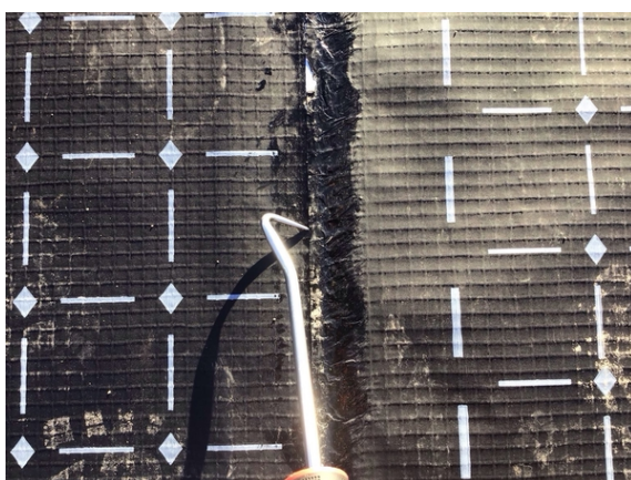
Testing hand welded membrane lap joint
