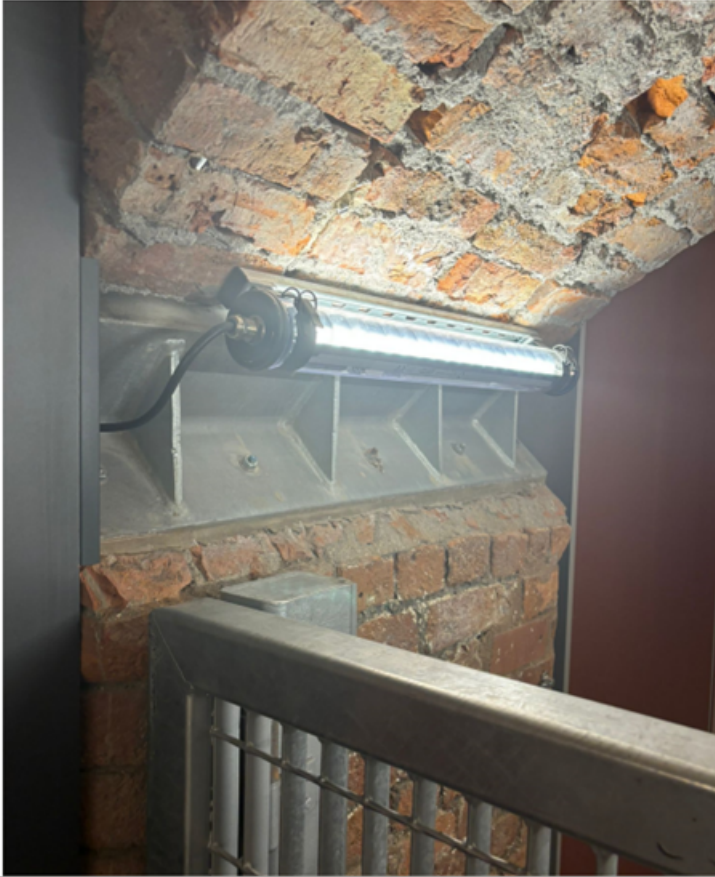
Figure 4 Arch Finishes at Spring Joints (Condition 4) (Project team's own photo)
