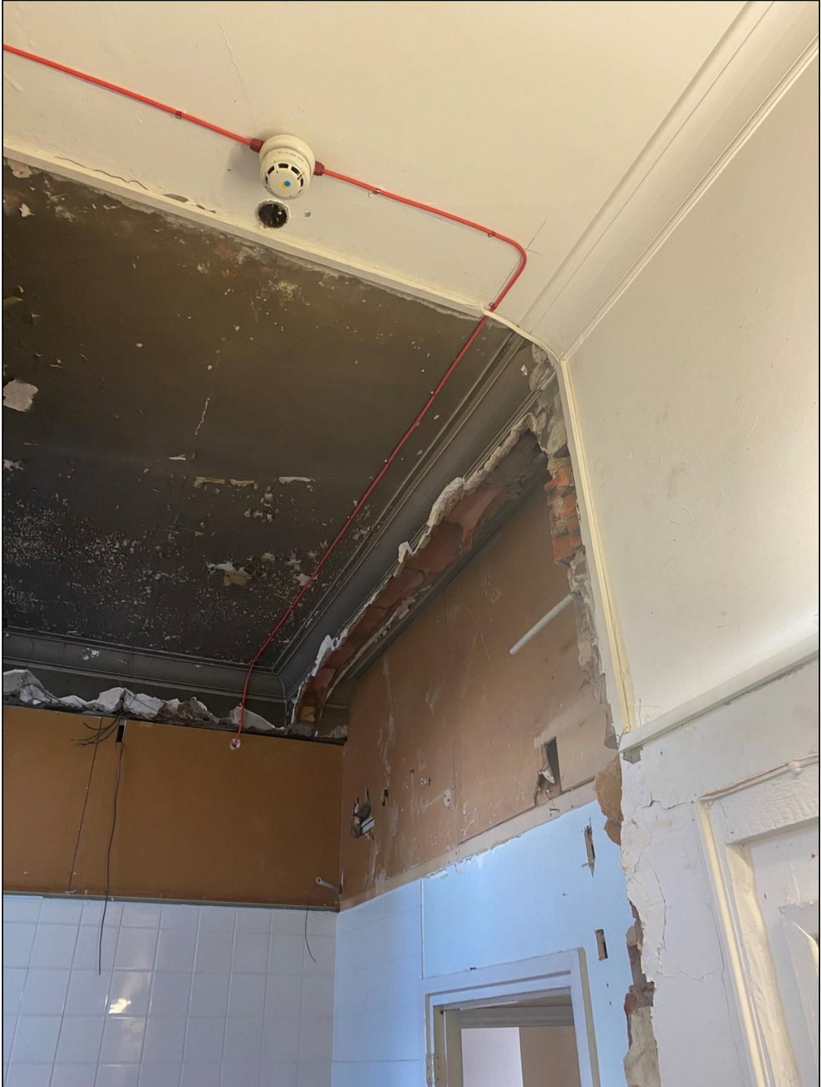
Caretaker's flat showing original position of wall
