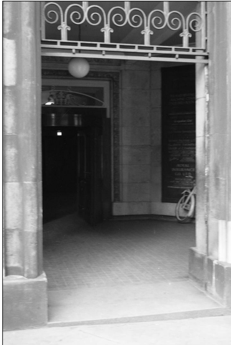
Figure 31 - Photograph dating to 1958, showing the original lobby.
