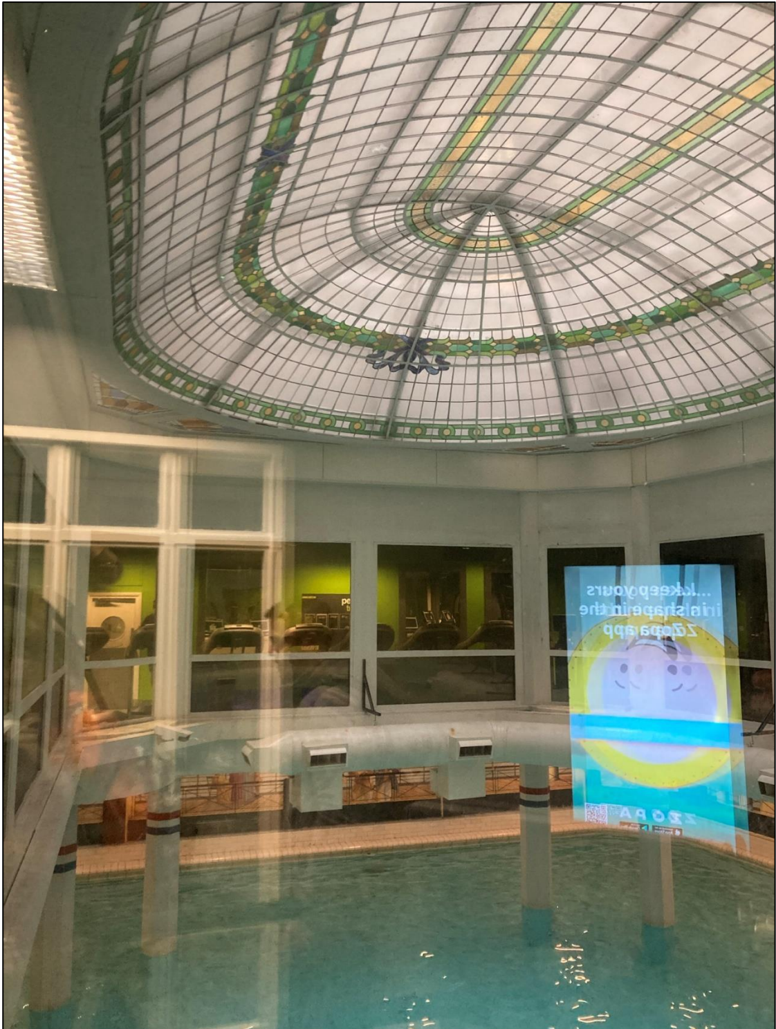
Existing pool with glazed dome above
