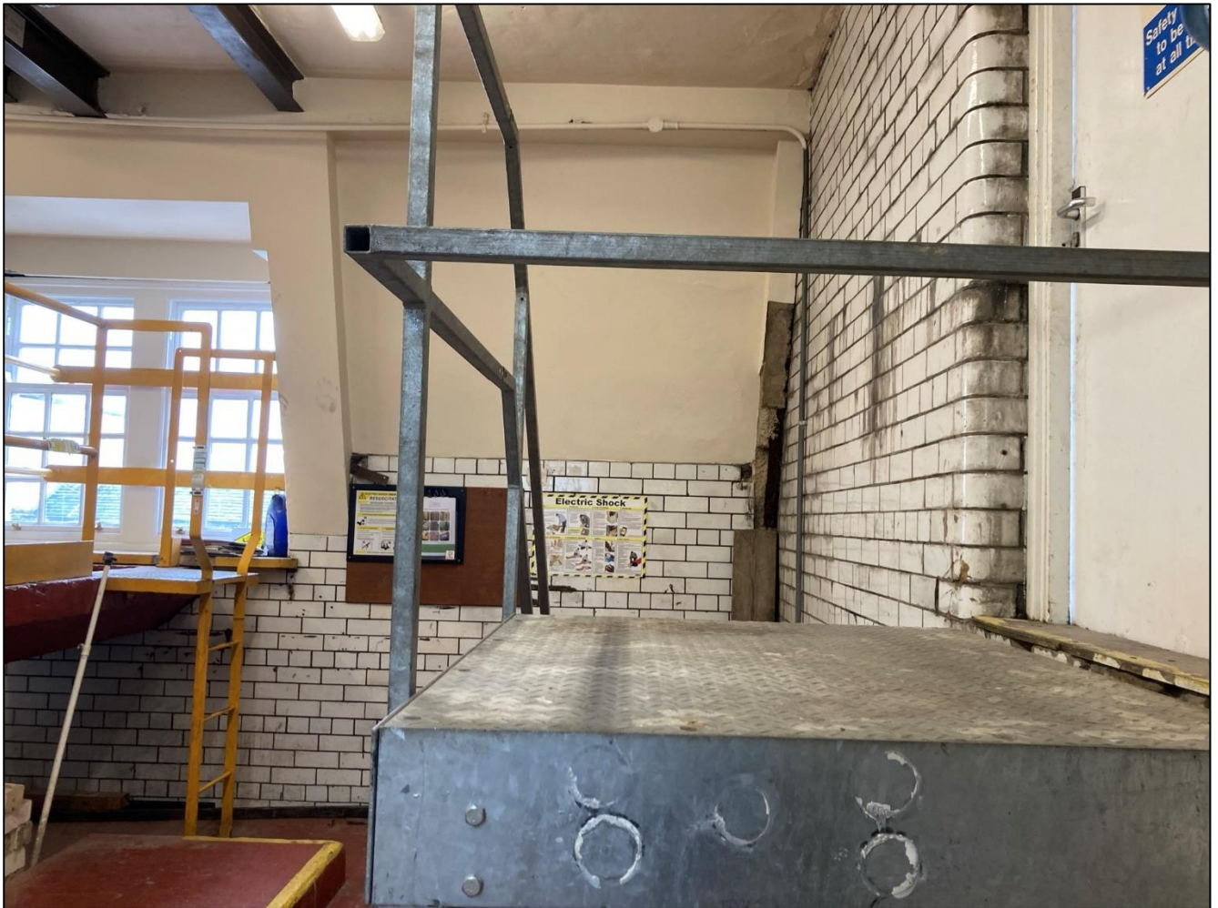
Lift motor room
