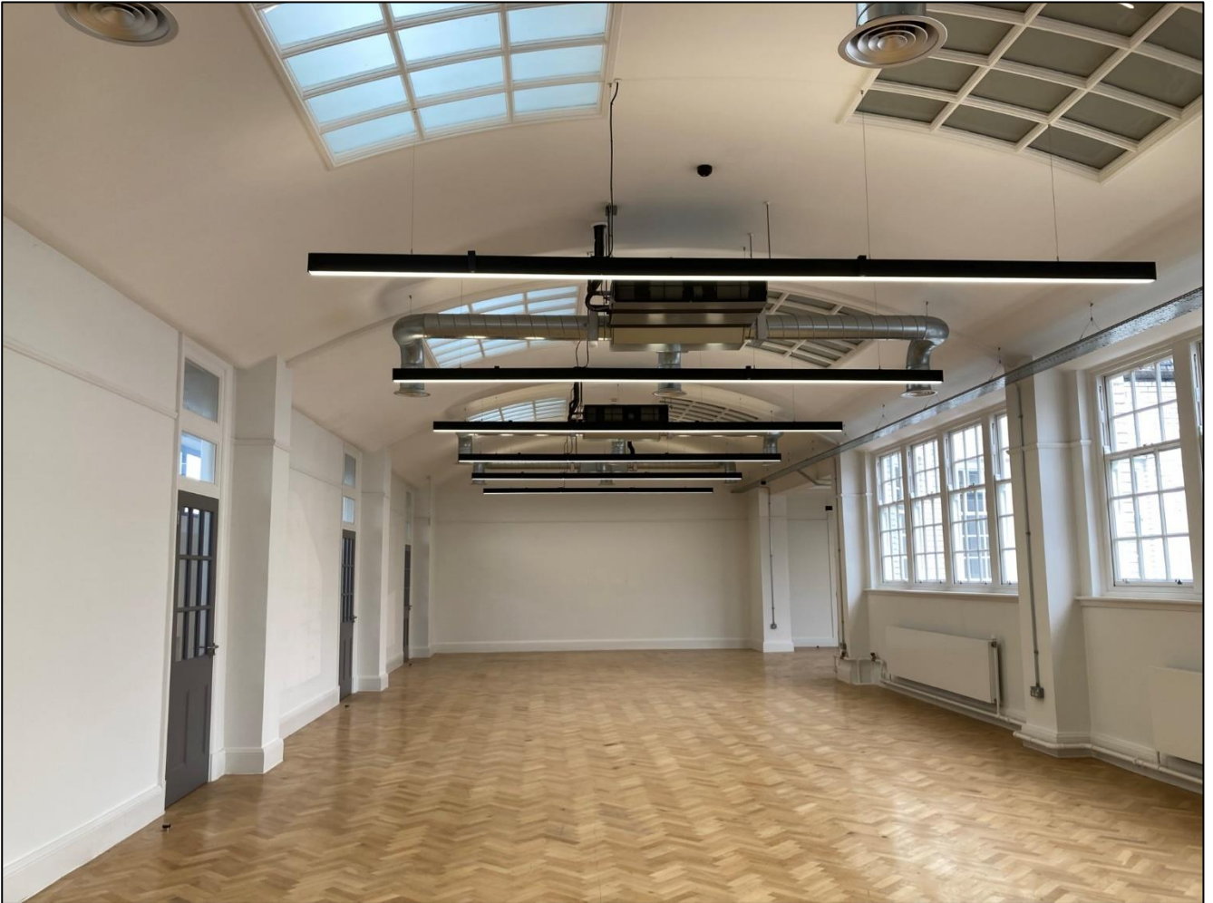
Original barrel ceiling with blocked up roof lights, thirteenth floor; wall nibs and doors denote original partitions
