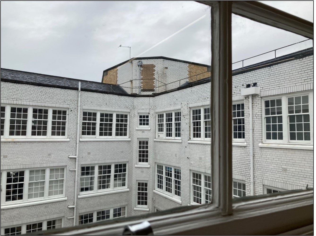
View into lightwell from the thirteenth floor
