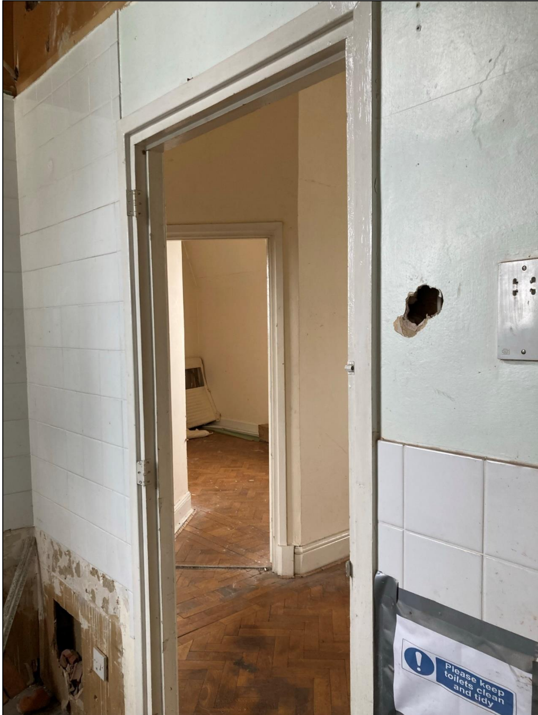
Original parquet flooring, caretaker's flat
