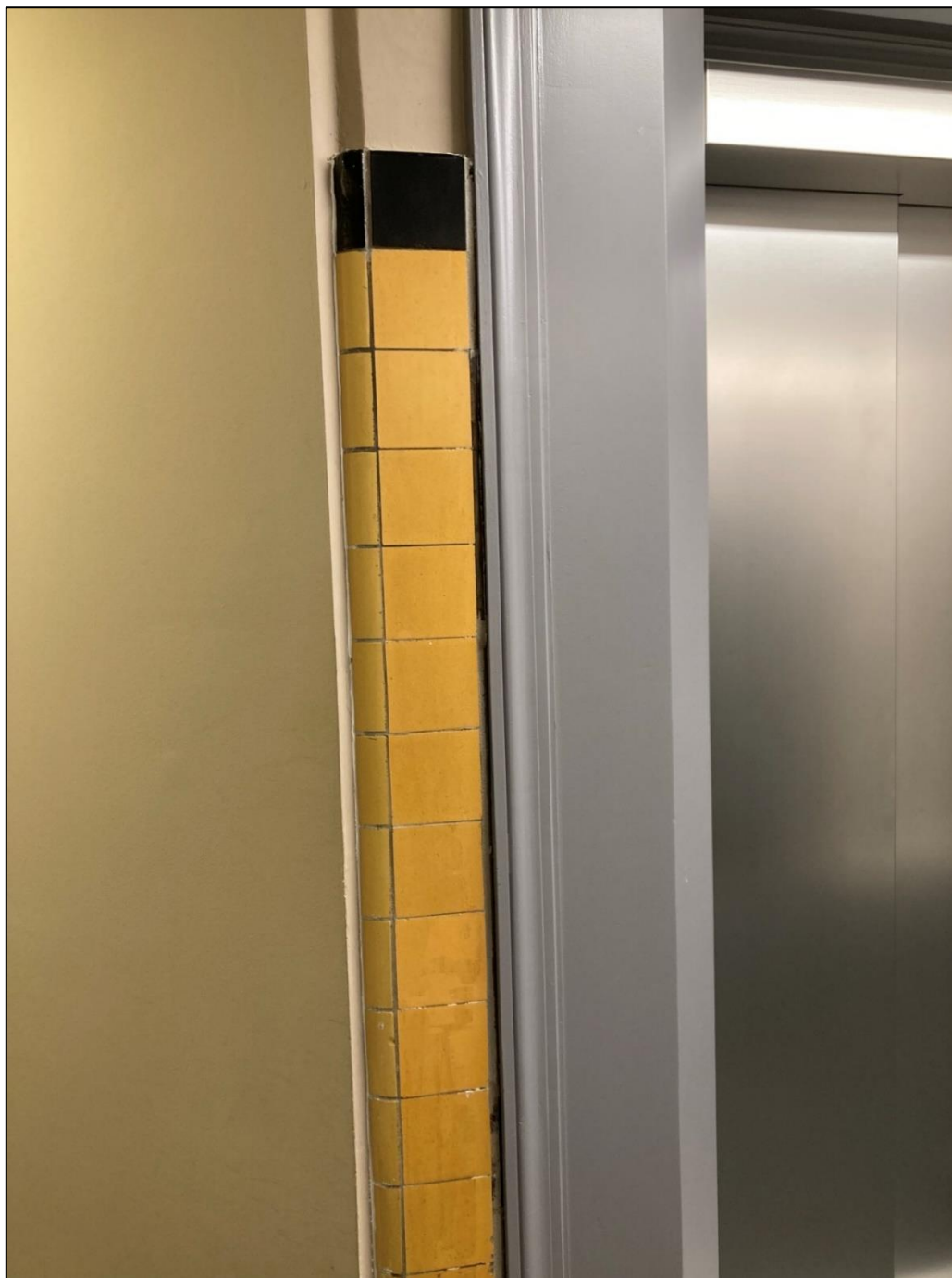
Original tiling adjacent to lift
