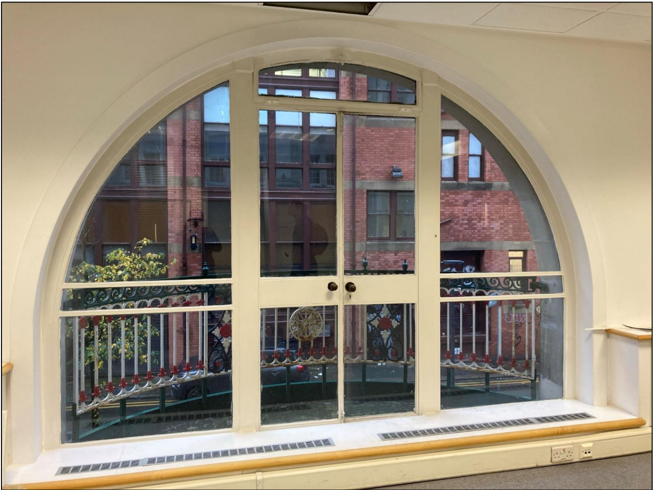
Existing balcony to first floor (onto Little Quay Street)
