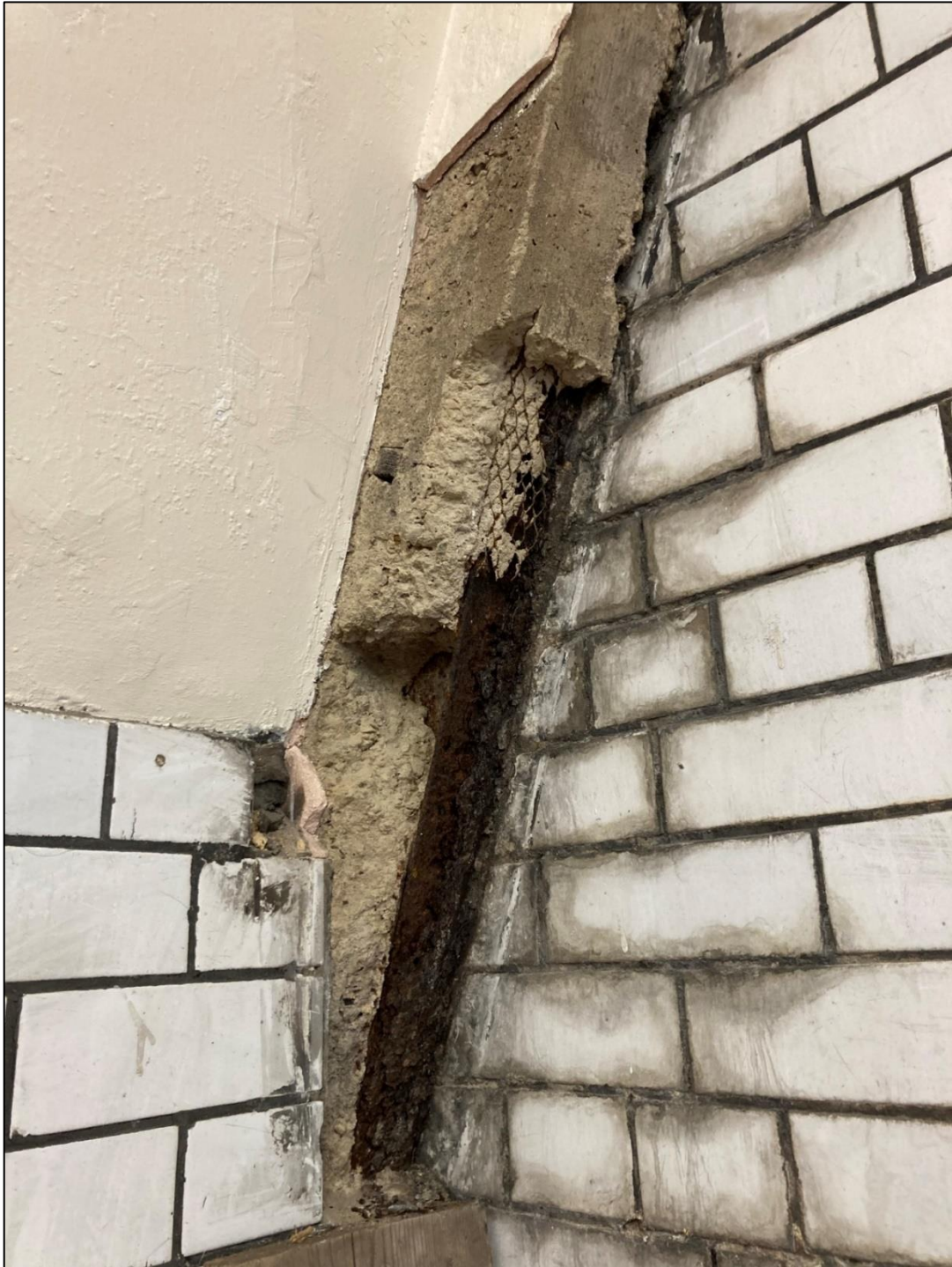
Exposed original wall construction in lift motor room
