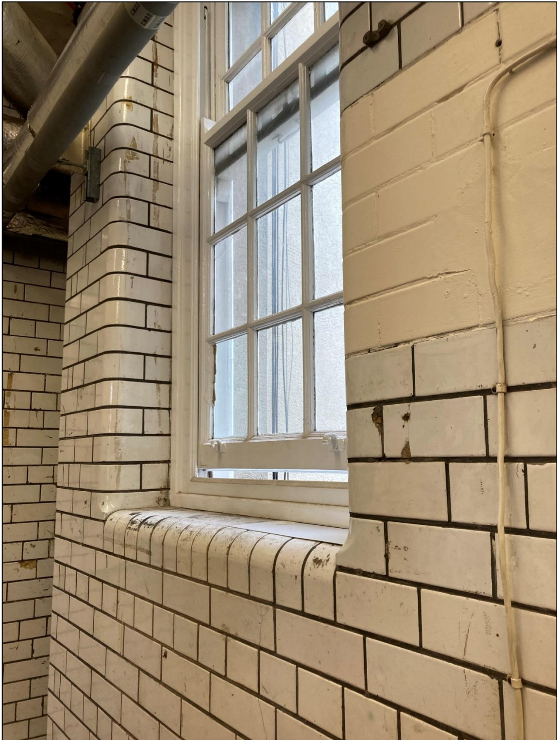
Original tiling within lift motor room
