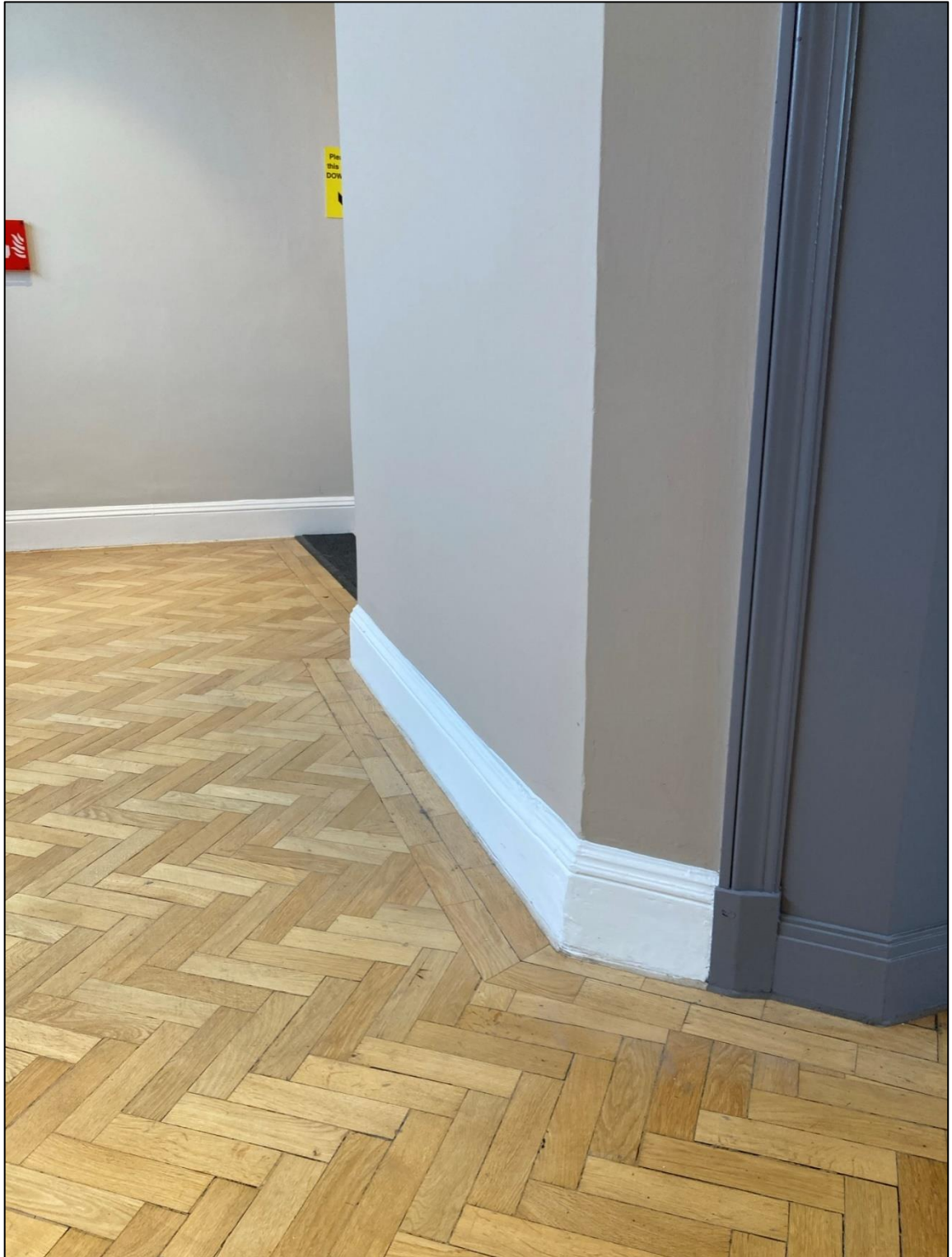
Original parquet flooring and skirting, thirteenth floor
