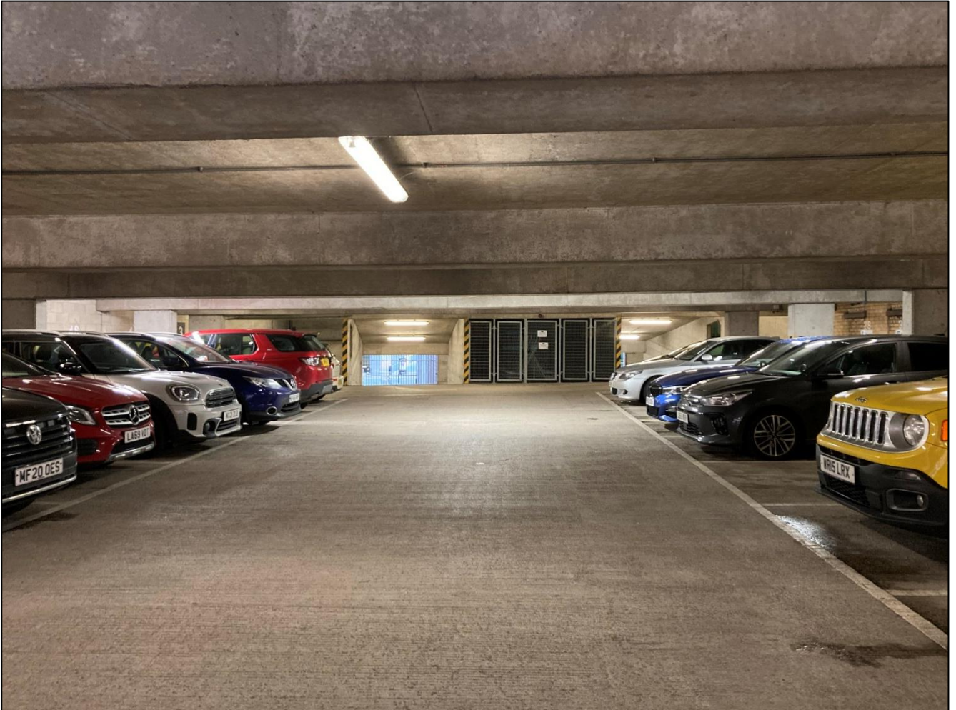
Interior of multi-storey car park
