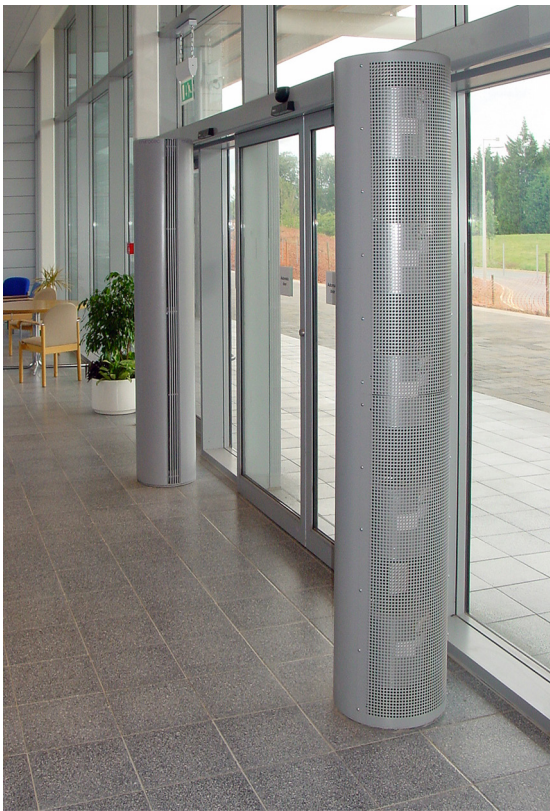
A pair of VCAC 2200/380 units with internal base plate.
