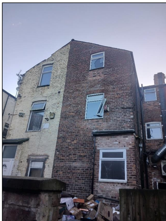
Figure 3: View of the rear of 430A Wilbraham Road (left) and 432A Wilbraham Road (right).
