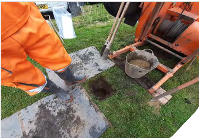
Photo 01: Hand dug service pit at CP04
