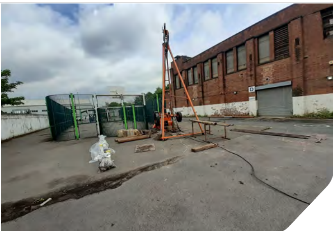
Photo 02: Cable Percussive Rig over CP02
