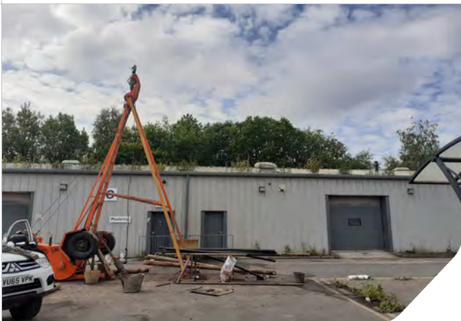
Photo 03: Cable Percussive Rig over CP03
