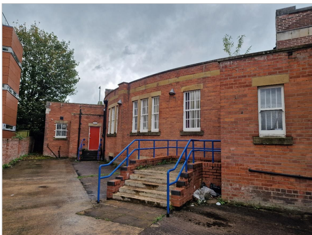
Figure 4.8: Sash windows to the north east rear elevation
