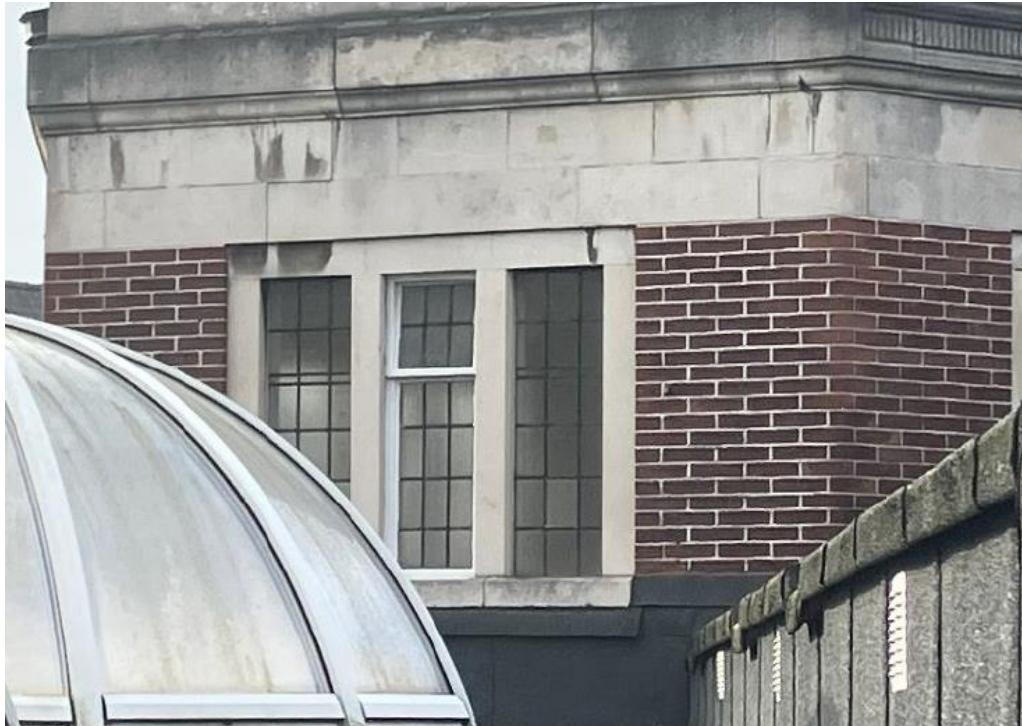
Figure 4.9: Leaded windows within crittall frames on the rotunda
