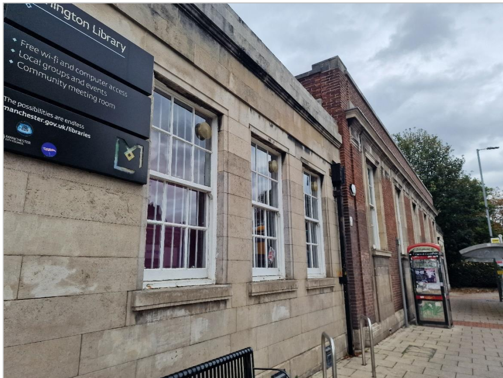
Figure 4.7: Sash windows to the south east elevation
