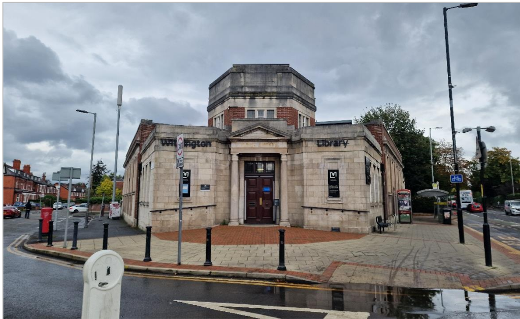
Figure 3.5: View north east of Withington Library from Wilmslow Road
