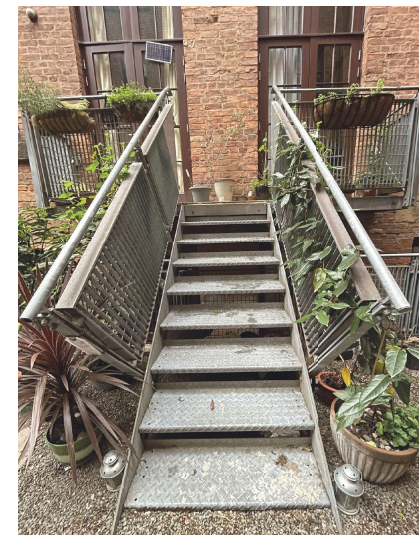
Fig. 06 Photo of existing aluminium checker plate stair treads.
