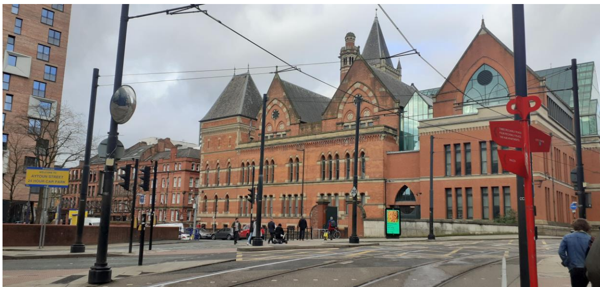
Plate 9: View looking NW from Piccadilly Place across Aytoun Street towards the S-facing elevation of the Crown Court with the car park visible to left of picture
