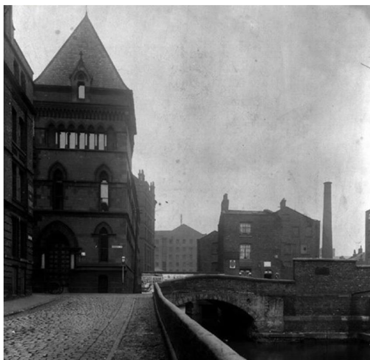
Plate A: View looking E from the Rochdale Canal towpath towards the Minshull Street, with the site visible to right of picture and the City Police Courts to the left
