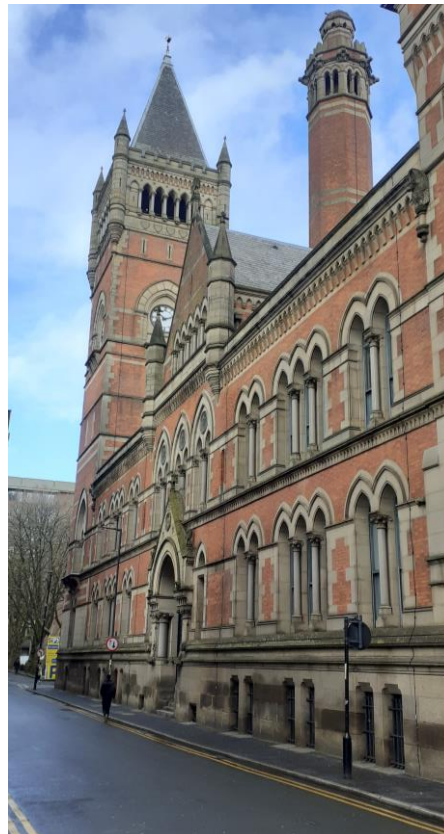
Plate 13: View looking NNW along Minshull Street showing the W-facing elevation of the Crown Court
