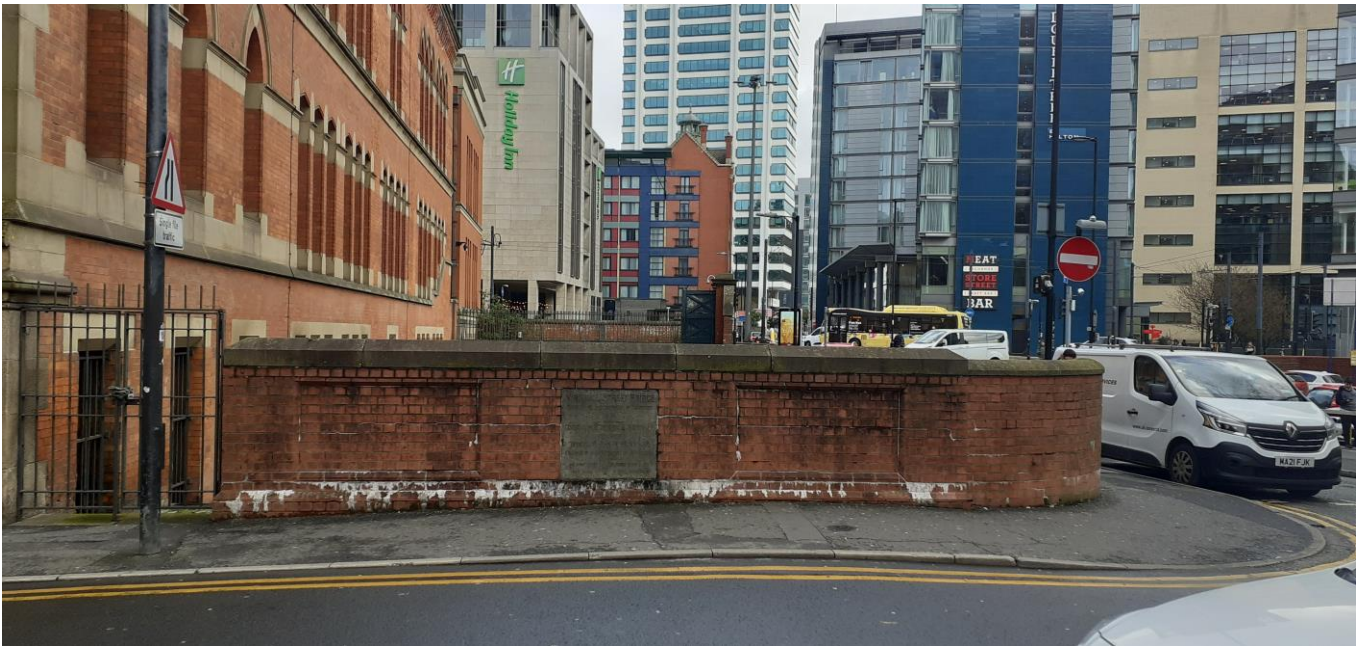
Plate 16: View looking NE towards Minshull Bridge across the Rochdale Canal (built in 1905), with car park to right of picture
