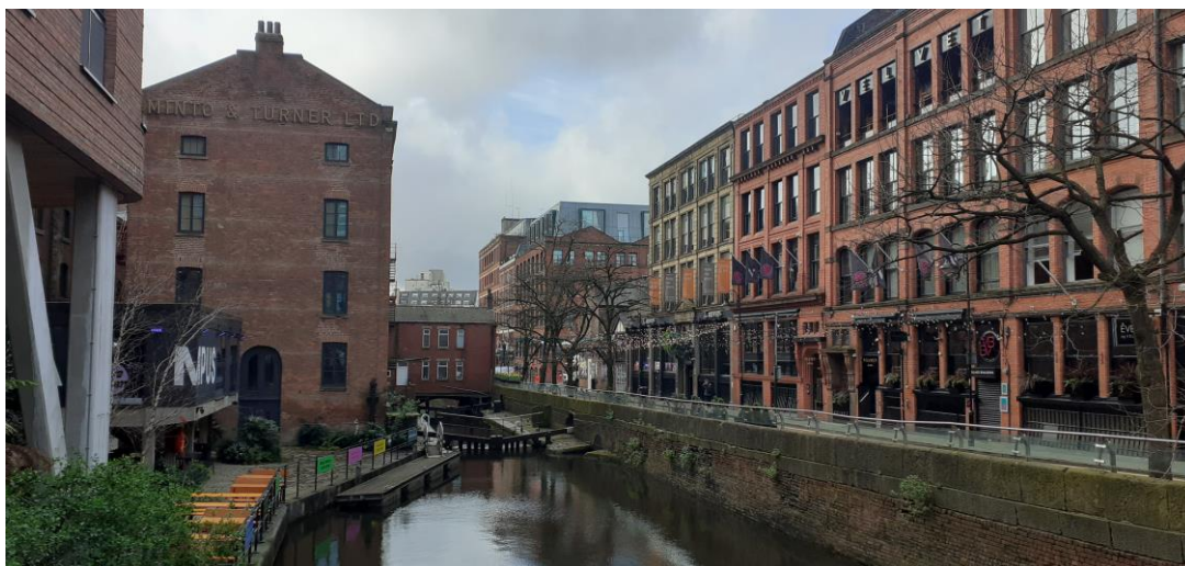
Plate 15: View looking SW from Minshull Street along the Rochdale Canal towards Lock 86 with the boundary wall running along Canal Street to right of picture
