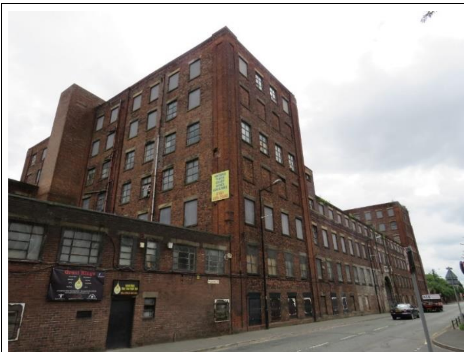
Figure 1 – The principal entrance front of the Mill as seen looking south-west along Bradford Road.
