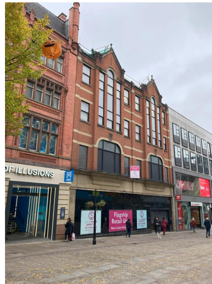
Fig. 1. Site location and immediate context
