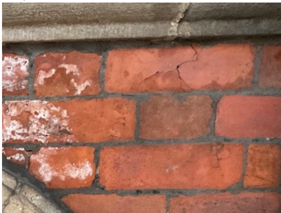
Existing pointing to brickwork is black ash mortar.
