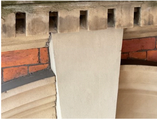
Existing and proposed indents (Johnson's Wellfield, Crosland Hill sandstone).
