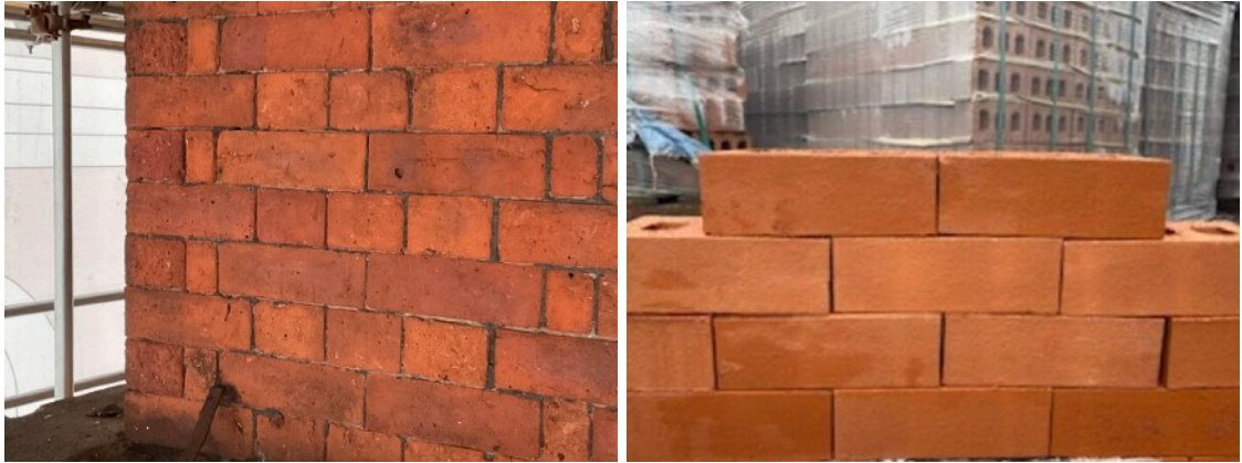
Existing and proposed bricks (Forterra St Anne's Smooth 75mm wirecut) or approved reclaimed.
