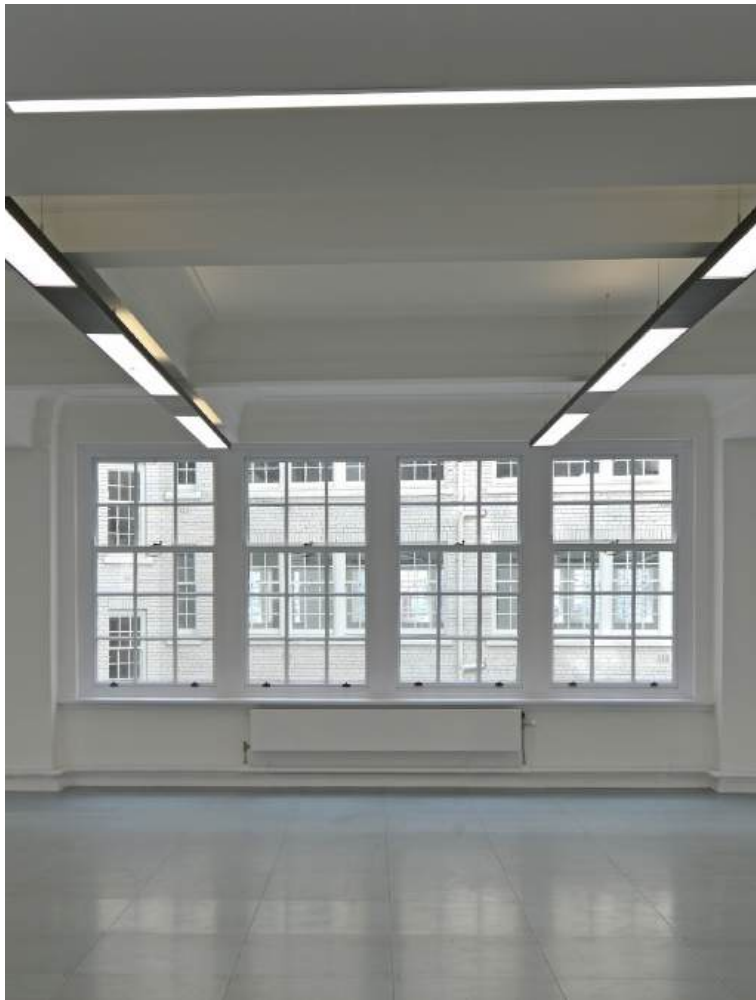
SASH WINDOWS TO LIGHTWELL AND OUTER FACADE
