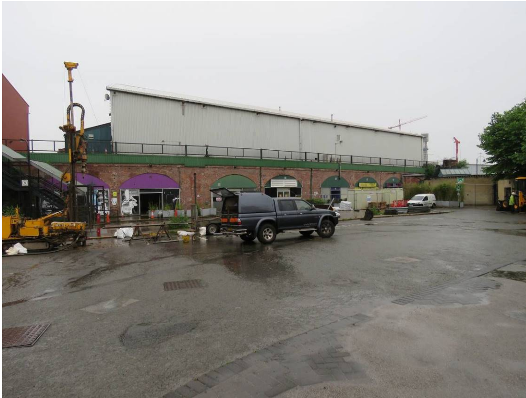
Figure 1A: photo of the brick arches and viaduct as it exists today; the former Starlight Theatre sits on top of the viaduct.
