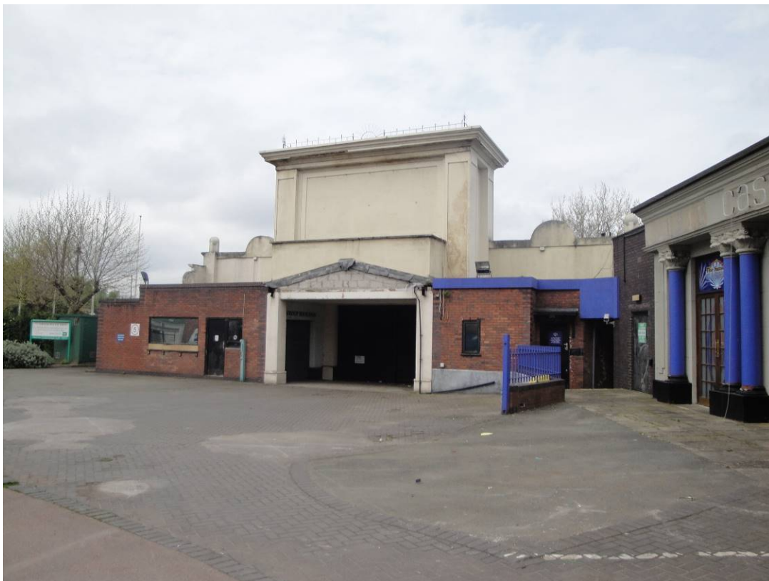
Figure 1B: photo of the former entrance into the site, from Water Street, and the former casino to the right. These structures will be demolished as part of the proposed development
