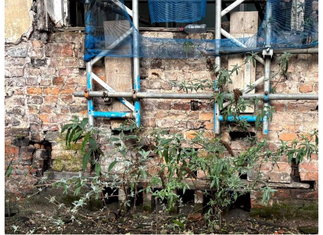
Joist pockets at ground floor level (January 2025)
