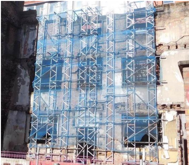
Internal elevation of façade (April 2023)
