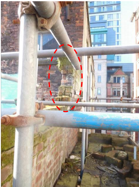
High section of wall at righthand end of façade (April 2023)
