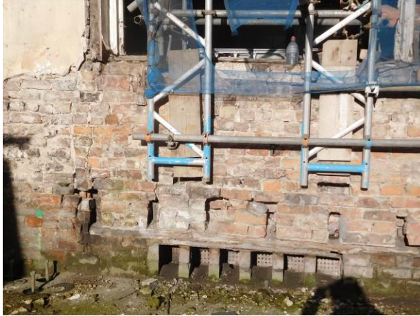
Joist pockets at ground floor level (April 2023)
