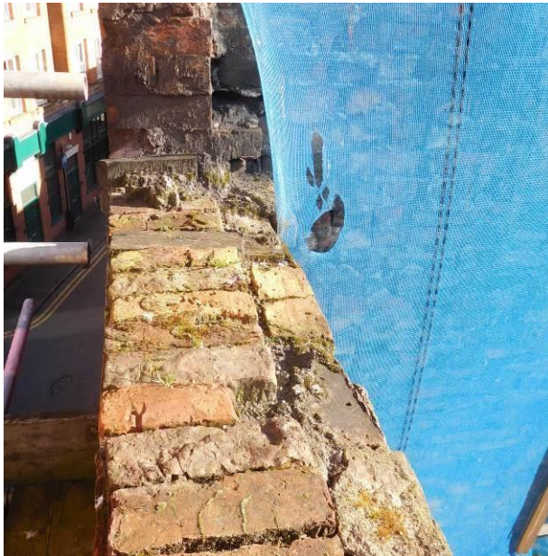
Typical brick on edge detail where present (April 2023)
