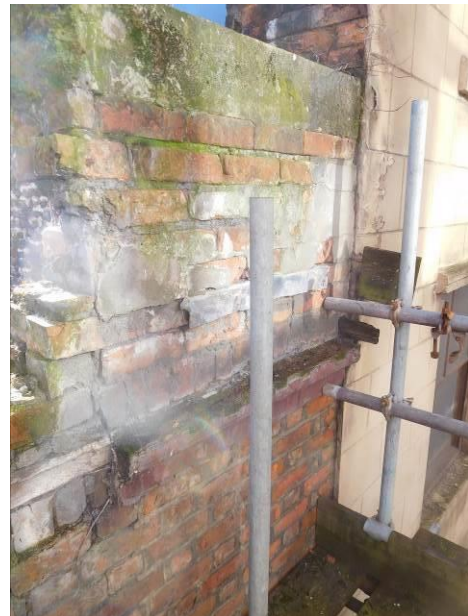
High section of wall at righthand end of façade (April 2023)
