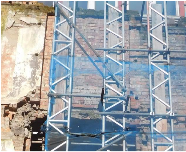
Brick infill on in situ concrete lintel (April 2023)
