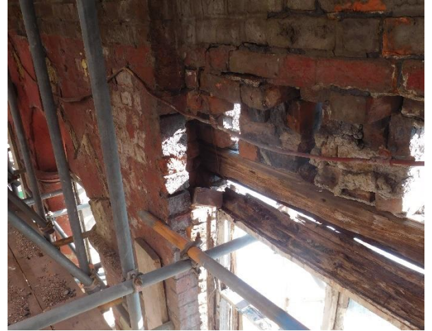
Joist pockets in wall (April 2023)
