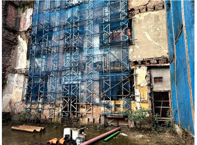
Internal elevation of façade (January 2025)
