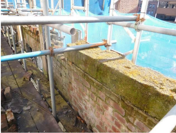
Concrete capping lintel to righthand end of wall (April 2023)
