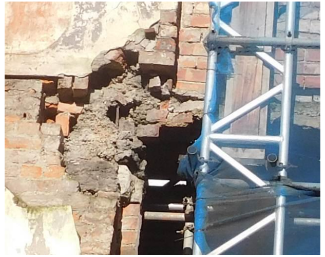
Detail of southern end of lintel (April 223)
