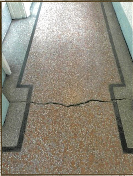
Large Crack to Corridor
