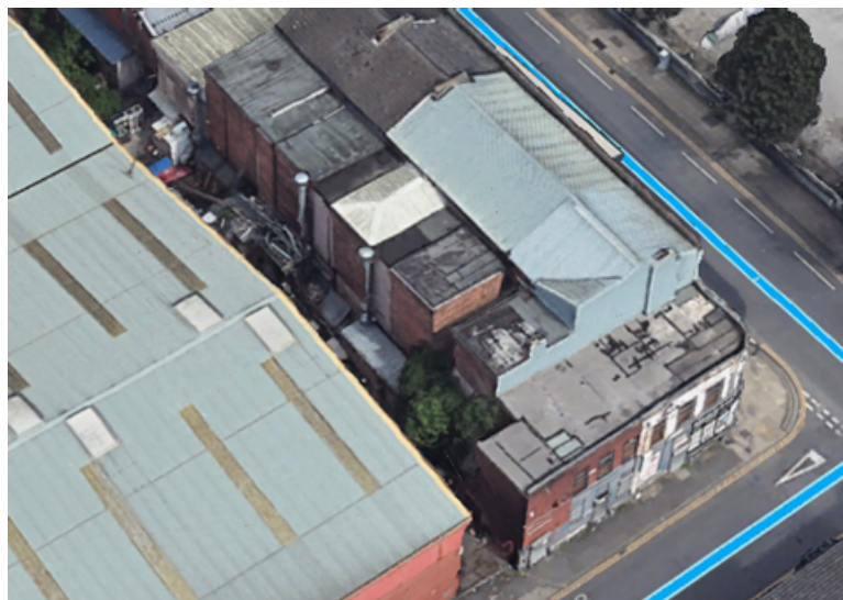
Fig. 4 – Aerial view of the application property
