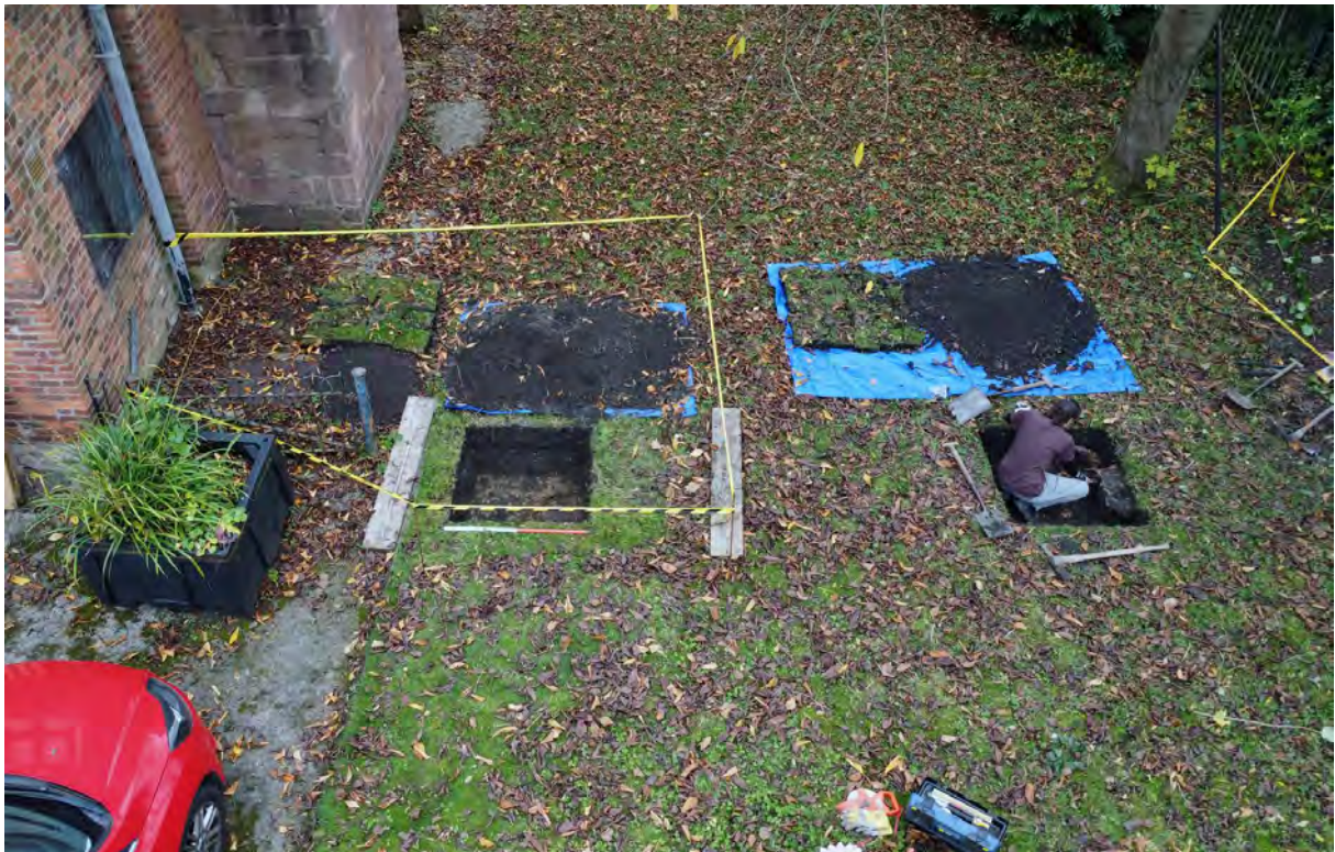
Plate 2. Trial pitting site, viewed from west, Trial Pits 1 (left) and 2 (right), under excavation.
