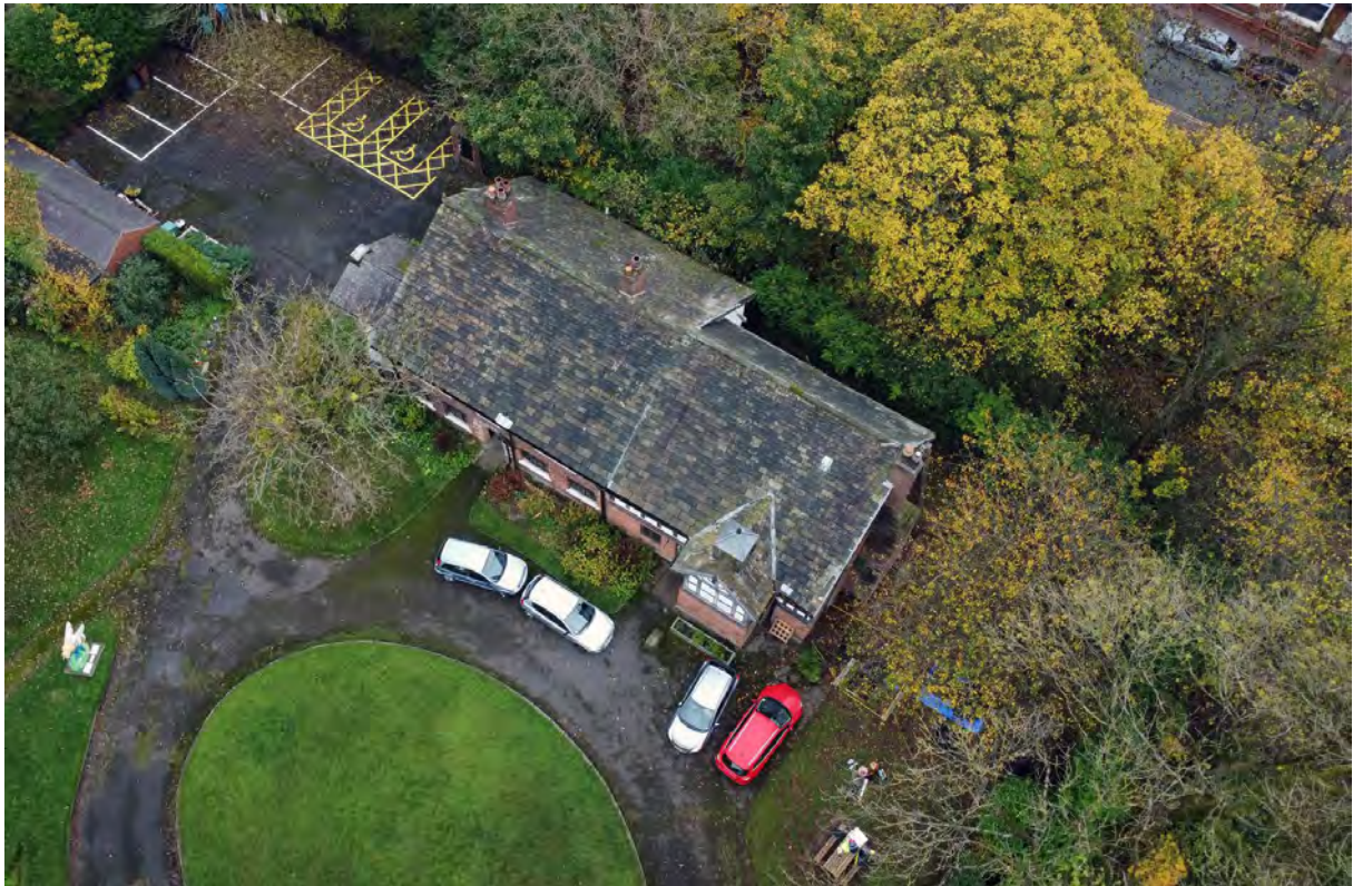
Plate 1. Clayton Hall, viewed from south-west, trial pitting site to lower right.
