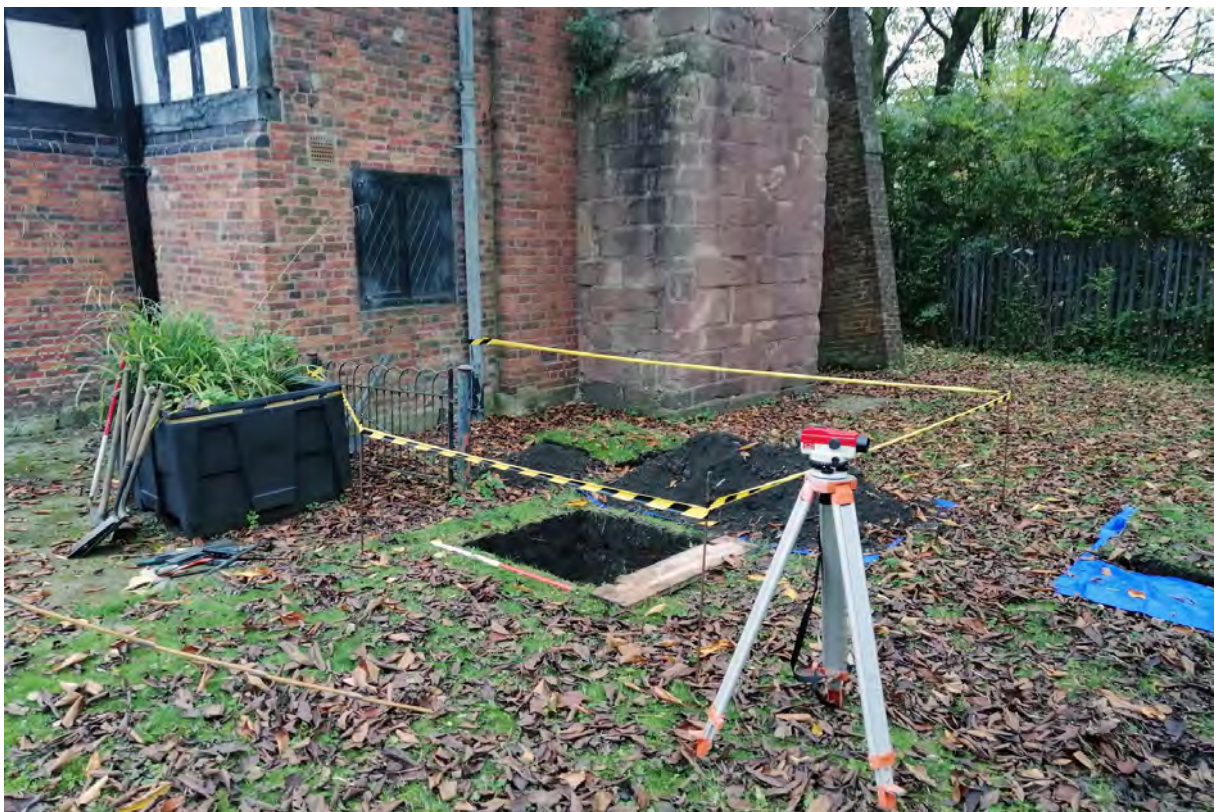
Plate 4. Trial Pit 1, viewed from south-west.
