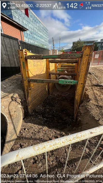
Plate 20: June 2 nd , re-enforced utility trench.
