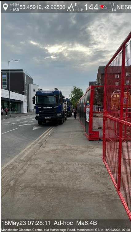
Plate 6: May 18 th , lorry outside site.
