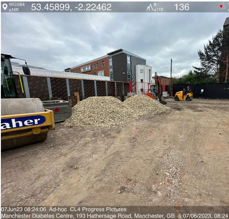
Plate 22: June 7 th , stone stockpile.
