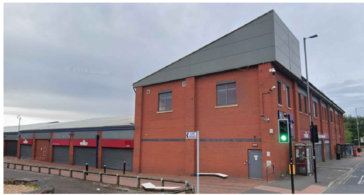
PHOTO OF ELEVATION AS EXISTING
