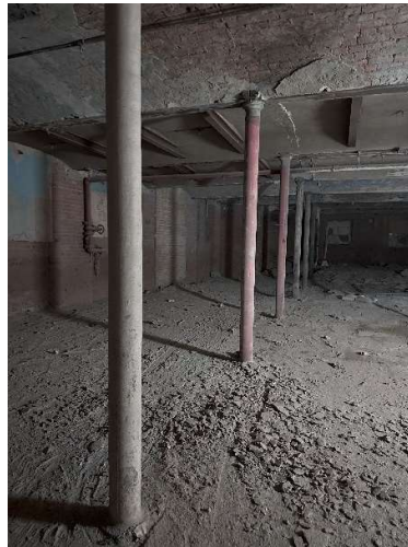
Figures 59 & 60. The ground floor, Bradford Road, previously masonry-encased columns, and paint remnants were just dusted when sample 16 was sought.
