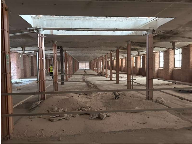
Figures 57 & 58: First-floor, main canal-side mill with columns strengthened and encased with later steel. No sample 15 could be taken.
