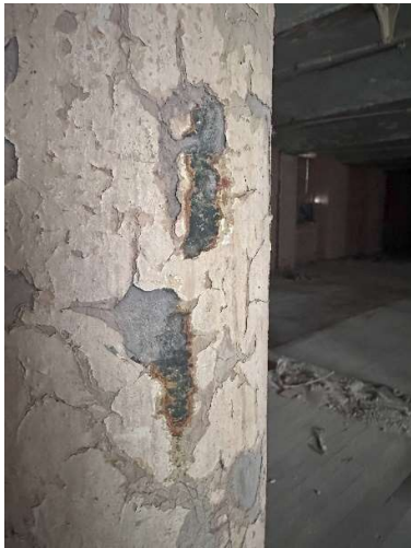
Figures 43 & 44. Sample 10 could not be taken as the earlier paints under the modern layer were badly deteriorated.
