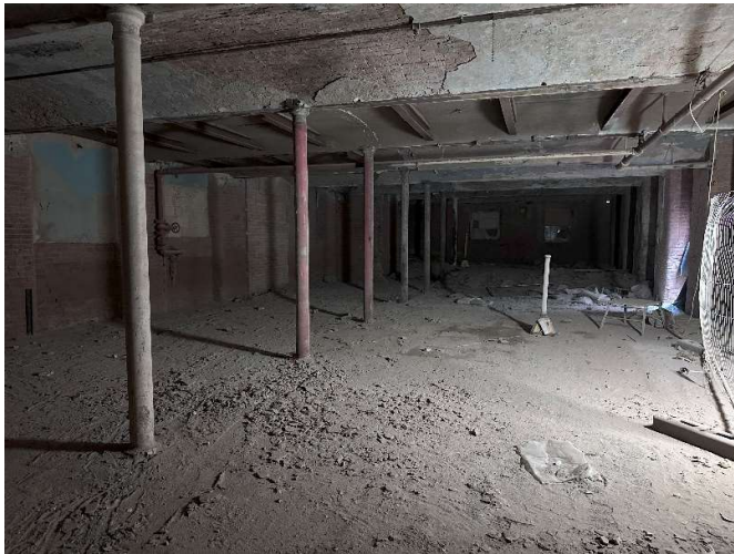
Figures 59 & 60. The ground floor, Bradford Road, previously masonry-encased columns, and paint remnants were just dusted when sample 16 was sought.
