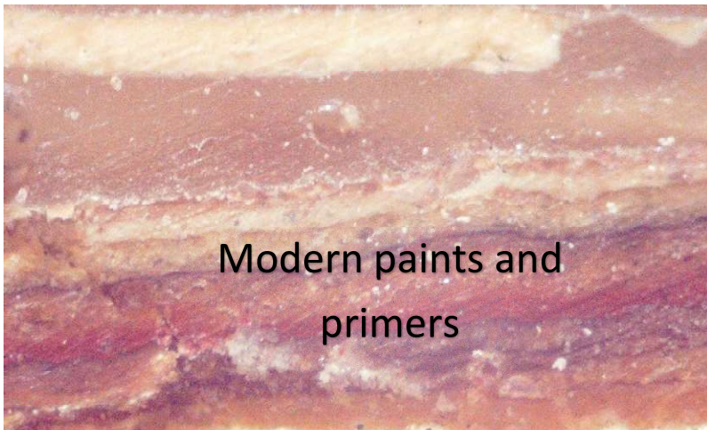
Figure 51. Second-floor, canal side. Sample 12 at X40
