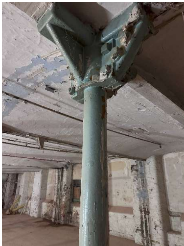
Figure 55. First-floor, south wing. Sample 13 was only modern paints.
