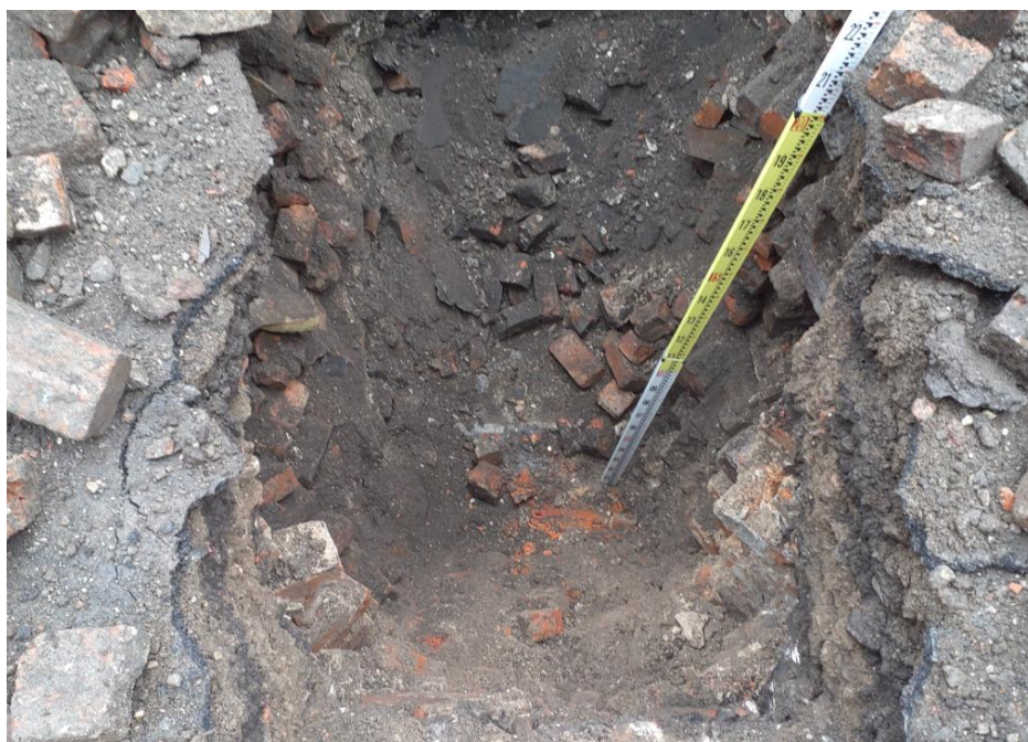
TP03 – Concrete Slab
