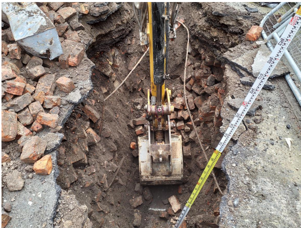
TP02 – Concrete Slab
