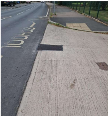
Photo 7: Tarmac patch repair to concrete access road.
