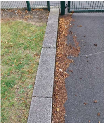
Photo 4: Concrete edging to pedestrian access path.
