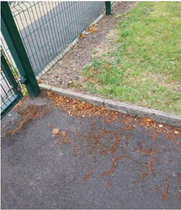
Photo 2: Concrete kerb edgings, no signs of damage.
