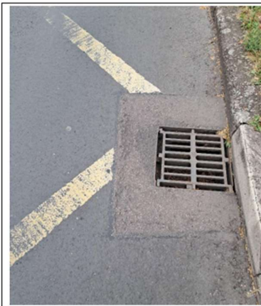
Photo 28 - Uneven kerb edgings to pedestrian path. Faded road markings.
