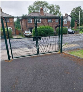
Photo 1: General view of main entrance to proposed contractors access to site. No visible defects.
