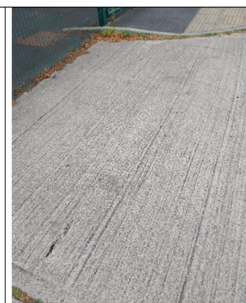
Photo 18 – Concrete access path in reasonable condition.
