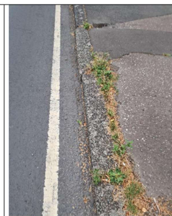
Photo 15: Generally uneven footpath surface course and kerb edgings.
