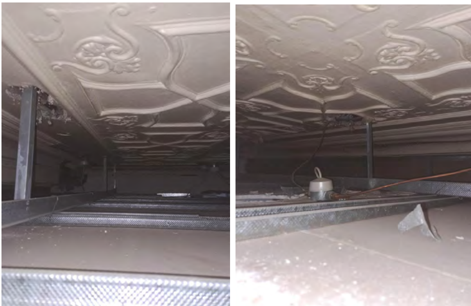
Figure 08: Images within ceiling void showing modern plasterboard support and holes existing holes in historic ceiling
