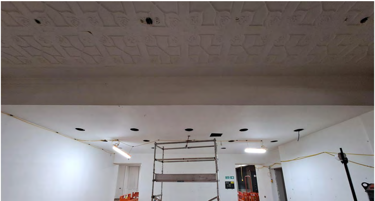
Figure 07: Existing modern plasterboard ceiling below decorative historic ceiling
