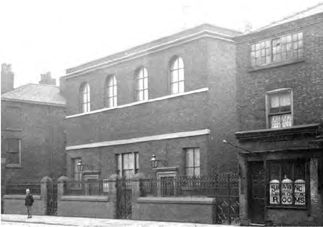
Figure 11: The south elevation of the c1823-4 chapel as seen in 1900, showing the replacement of the original sash windows with fixed windows (Source: Manchester Archives)
