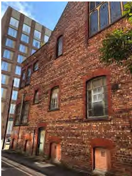
Figure 42: The rear, north elevation on Dyche Street.
