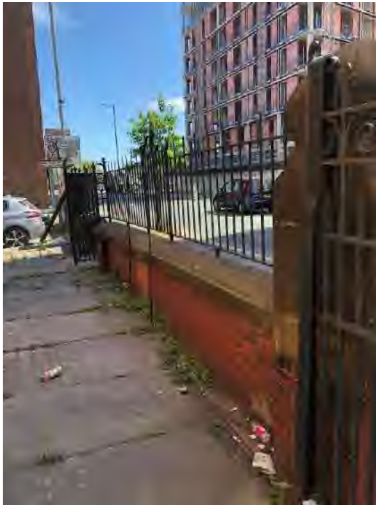
Figure 34: The eastern half of the reused 19 th century stone copings, gates and piers.
