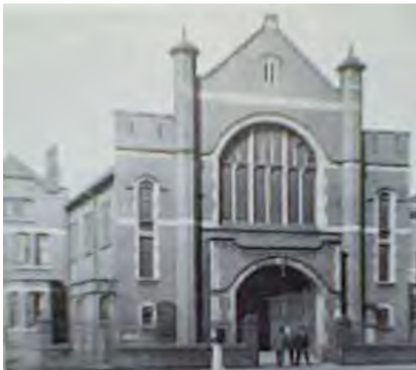
Figure 26: A view looking north-east, showing the western elevation of the chapel and original dwelling to the western side of the Site in c1960 (Source: http://freestgeorges.blogspot.com )
