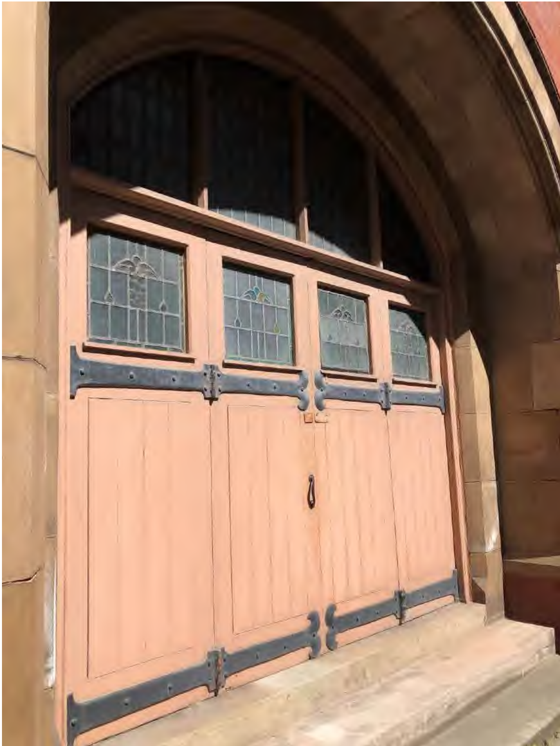
Figure 30: The original buff terracotta entrance portal, with concertina entrance doors that include an exemplar example of the Arts and Crafts style in the form of elongated metal hinges.
