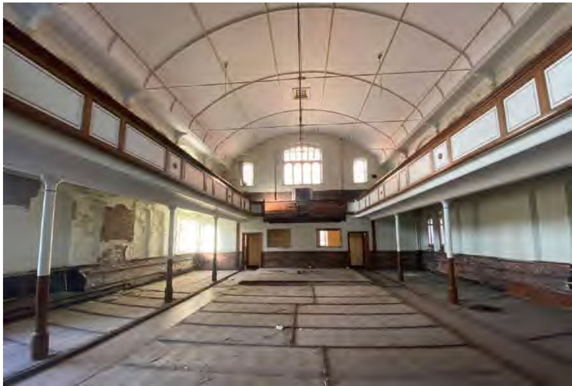
Figure 44: Looking north through the nave of the Chapel as it appears today, showing the balcony railings that were reused from the earlier Chapel.
