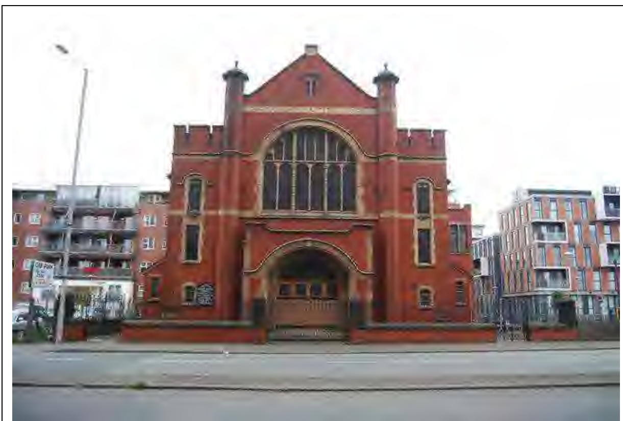
Figure 27: The principal south elevation, constructed from deep red brick and buff-coloured, unglazed terracotta. The retained earlier stone coping stones, gate piers and iron gates can be seen in the foreground.
