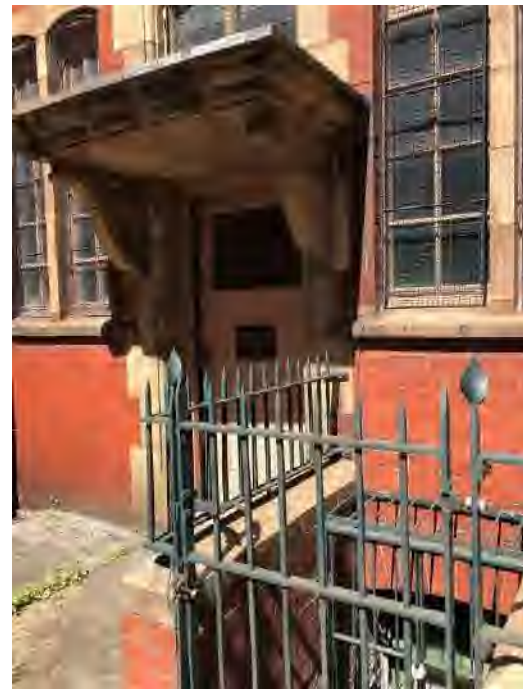
Figure 33: The original buff terracotta door canopy and Arts and Crafts metal basement railings.
