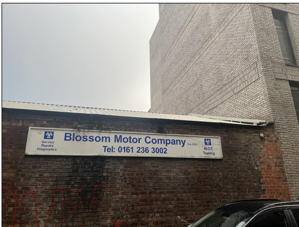
Plate 2 – Signage on north-eastern elevation, corrugated metal roof.
