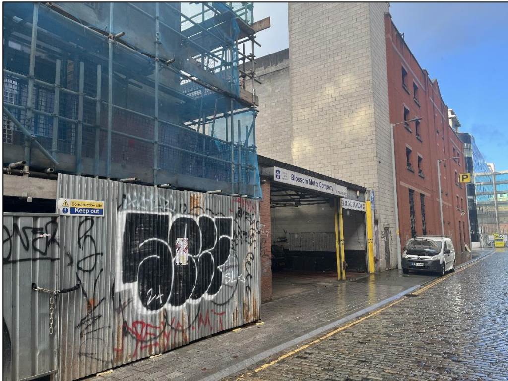
Plate 4 – Rear (north-east) elevation of site, with rolling shutter.
