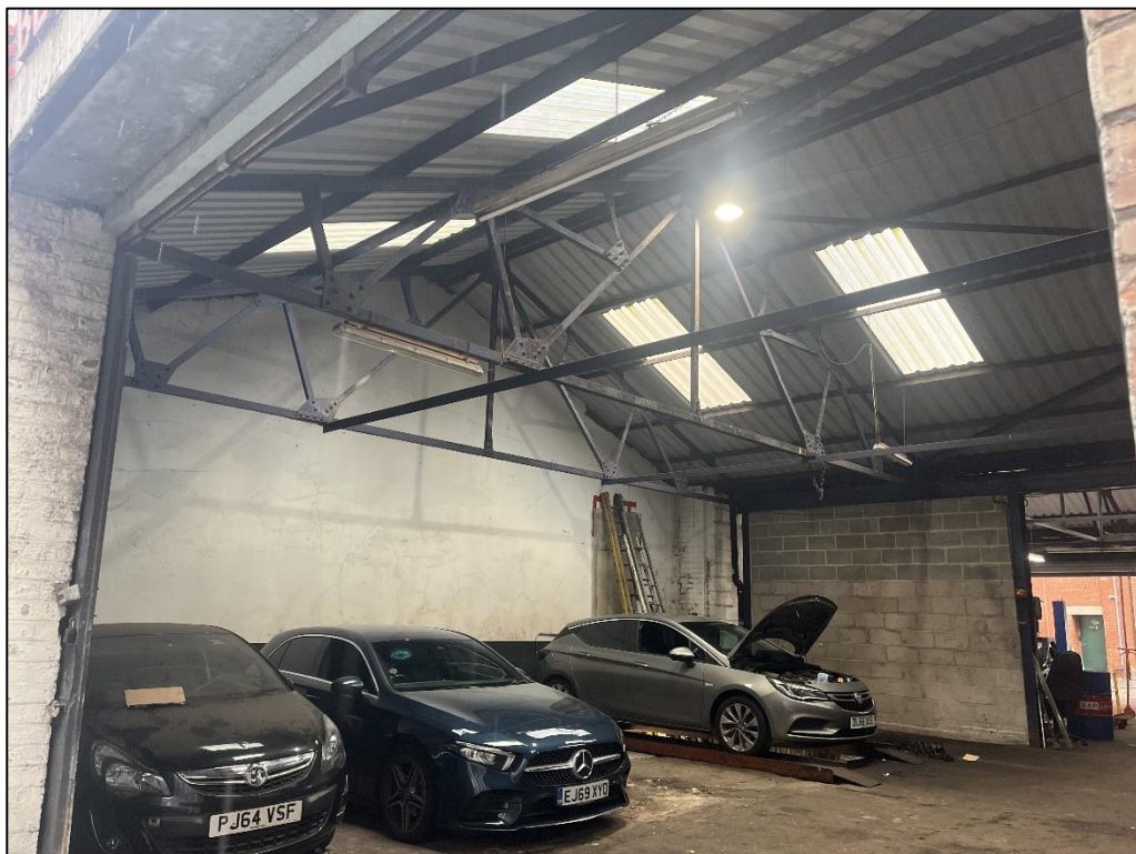
Plate 6 – Internal conditions of structure.
