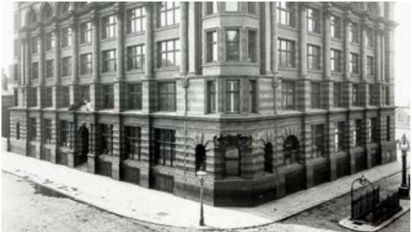
Image of building with original windows in place
