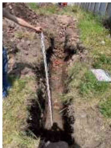
Trench 2: View of excavation
