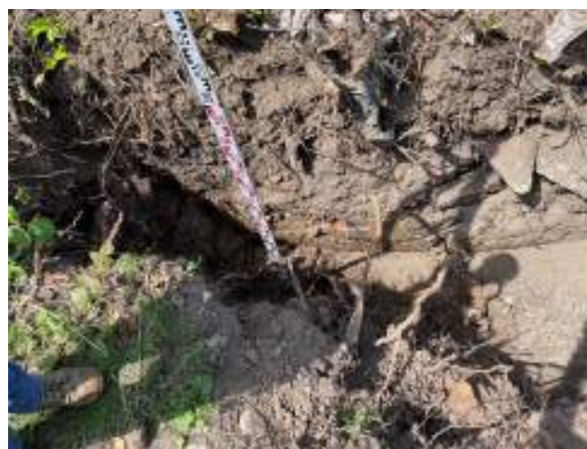
Pit B: View of excavation
