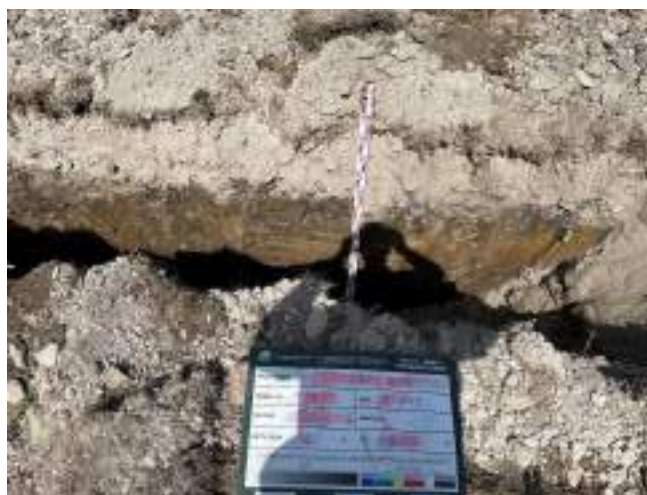
Trench 4: View of excavation
