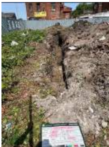
Trench 5D: View of excavation
