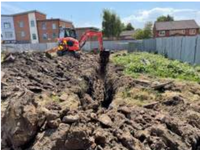
Trench 5A: View of excavation
