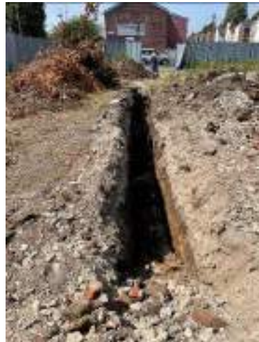
Trench 3: View of excavation
