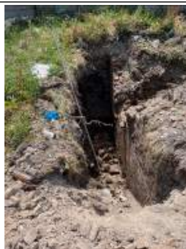
Pit C: View of excavation
