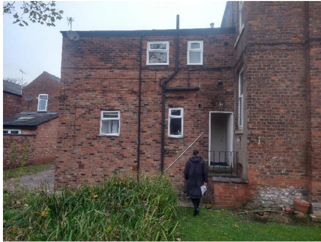
Figure 5. Existing Rear access up to outrigger-down to cellar
