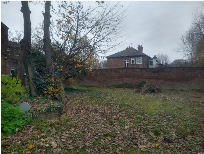
Figure 7. Gable to Moorfield Avenue
