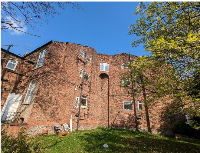
Figure 3. Gables to Nos 5&6
