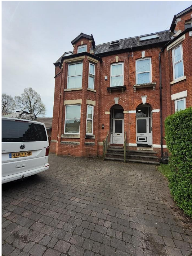
Figure 16. Beaconsfield South wing end
